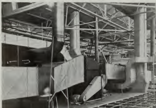
Two views of the heating and ventilating system in the paint department of the new plant of Vultee Aircraft, Inc., at Downey, Calif. Taken from opposite sides, they show the bell-driven motors, batteries of air filters, and parts of the huge gas furnaces.
