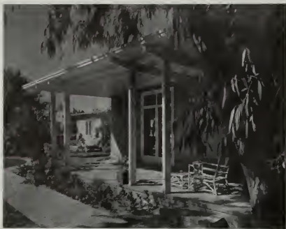
OPEN PORCH WITH ENTRANCE INTO THE LIVING ROOM
