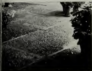
7 REDWOOD STRIPS AND CONCRETE
