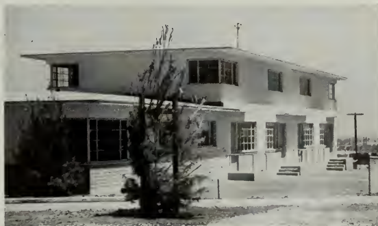
• Reginald D. Jahnson, Donald B. Parkinson, Eugene Weston, Jr., Lewis Eugene Wilson and A. C. Zimmerman, Architects. Howard Smits, Structural Engineer. Harvey Nichols, General Contractor. J. A. Powers, Mason Contractor.
