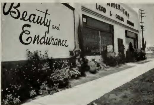
General Offices, American Lead & Color Works
