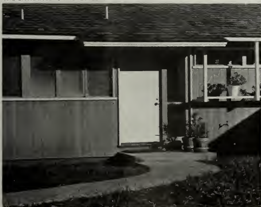
THE ENTRANCE IS PROTECTED BY AN EXTENDED EAVE
