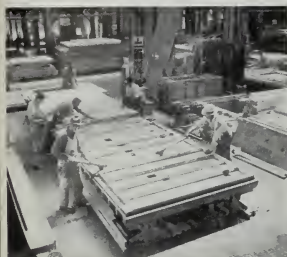
APPLYING GLUE TO WALL SECTIONS
