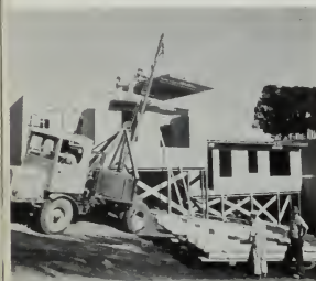
COMBINATION ROOF-CEILING SECTIONS
