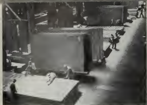
GENERAL VIEW OF THE SHOP
