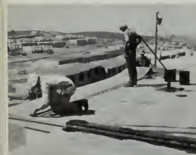
APPLYING BUILT-UP ROOFING
