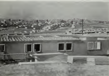
COMPLETED UNITS AT VALLEJO
