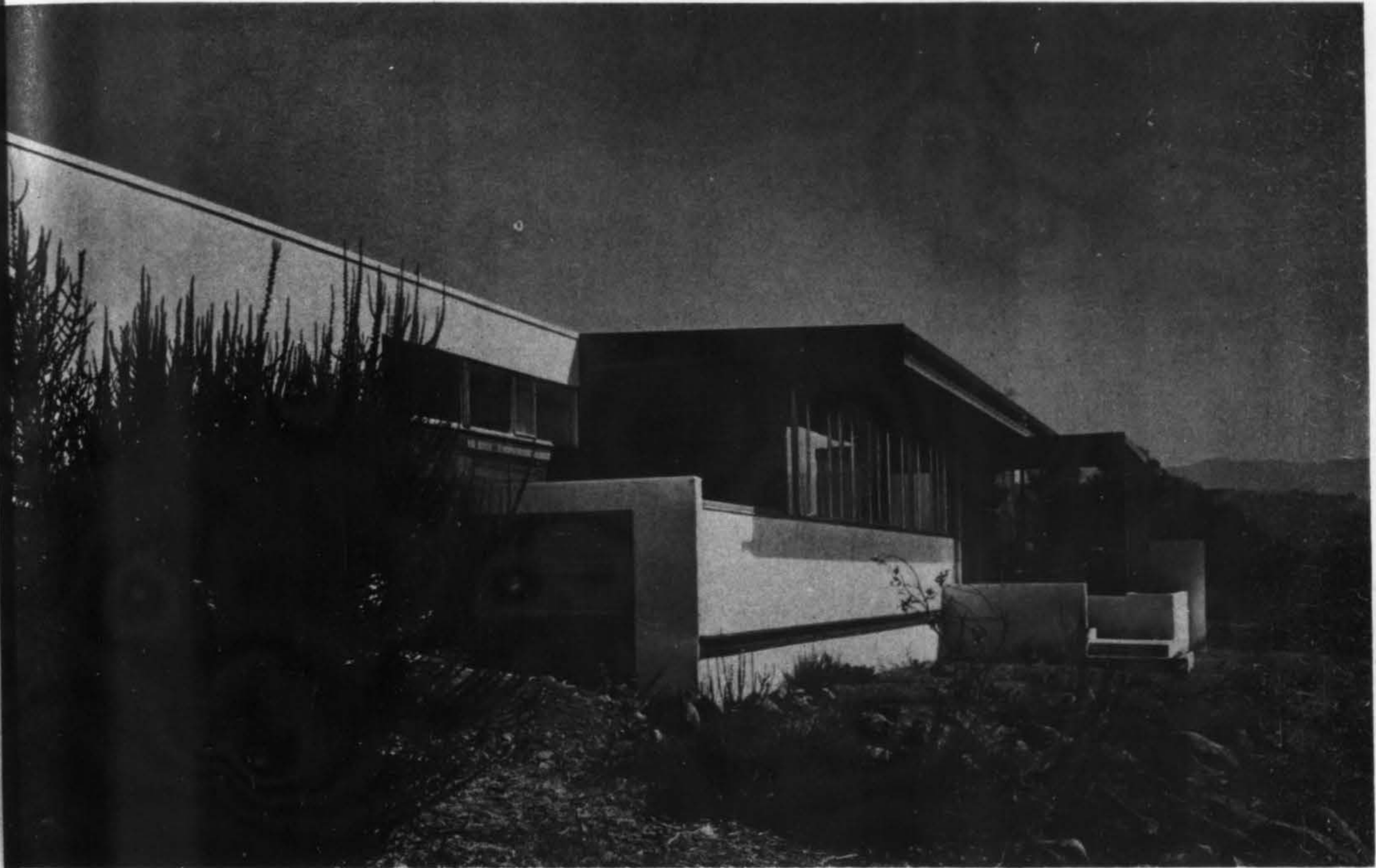
THE EXTERIOR IS OF NATURAL CALIFORNIA REDWOOD SIDING TREATED WITH SPAR VARNISH AND CEMENT PLASTER BRUSH-COATED OFF-WHITE
