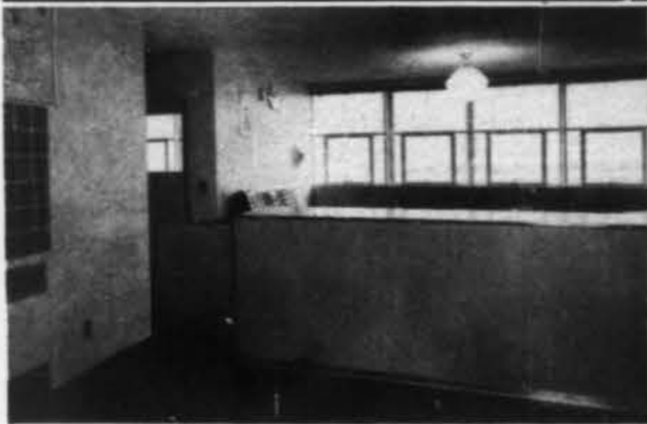
BOTH COUNTERS AND CUPBOARDS at Acalanes Union High are constructed of Douglas Fir Plywood, Plypanel grade. All plywood wall panels were butted together without battens.
