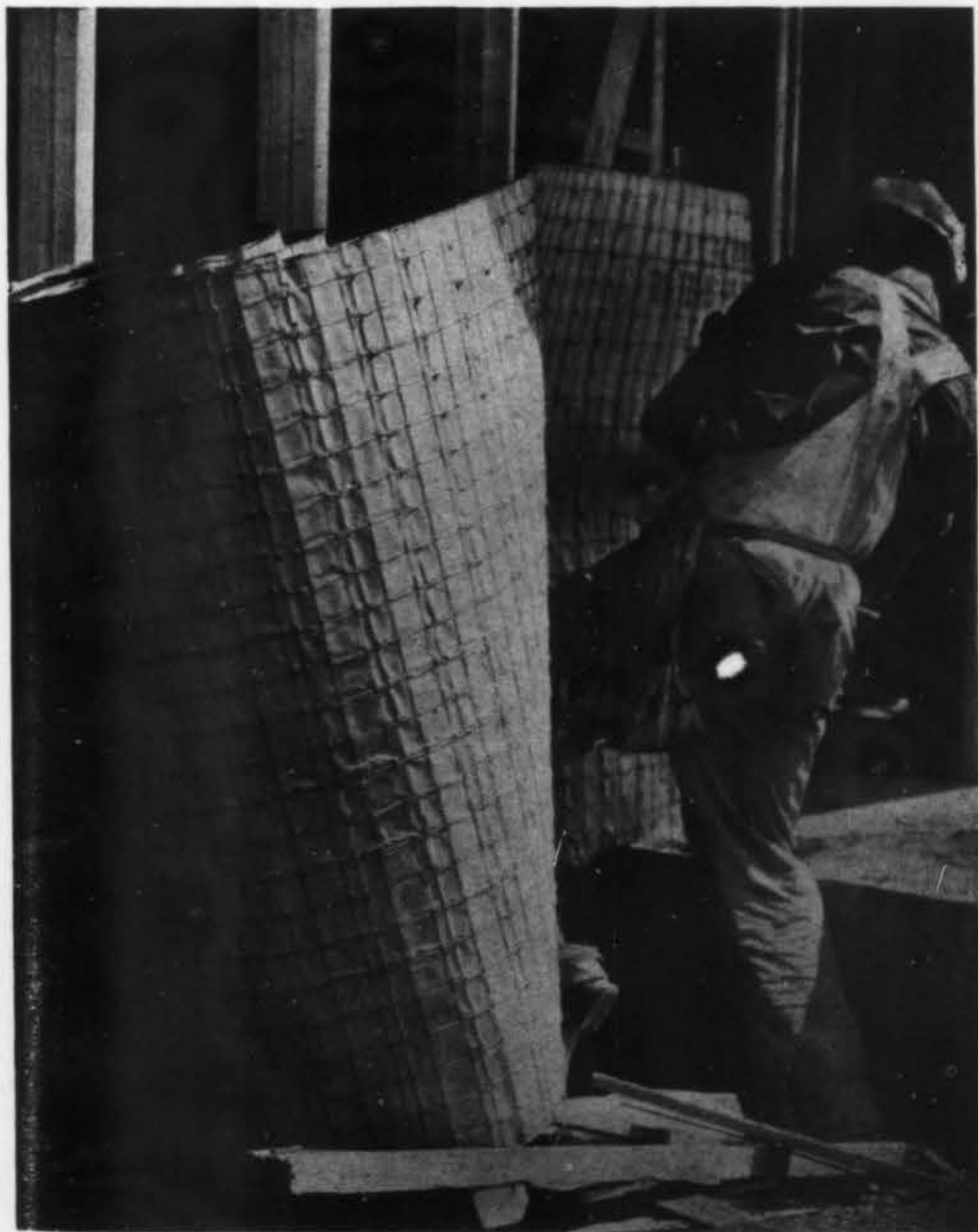
Steeltex Cuts Expense and Work at Avalon Gardens
