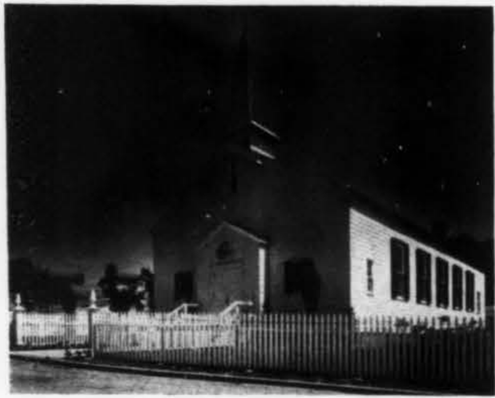
CHAPEL AT FORT MacARTHUR
