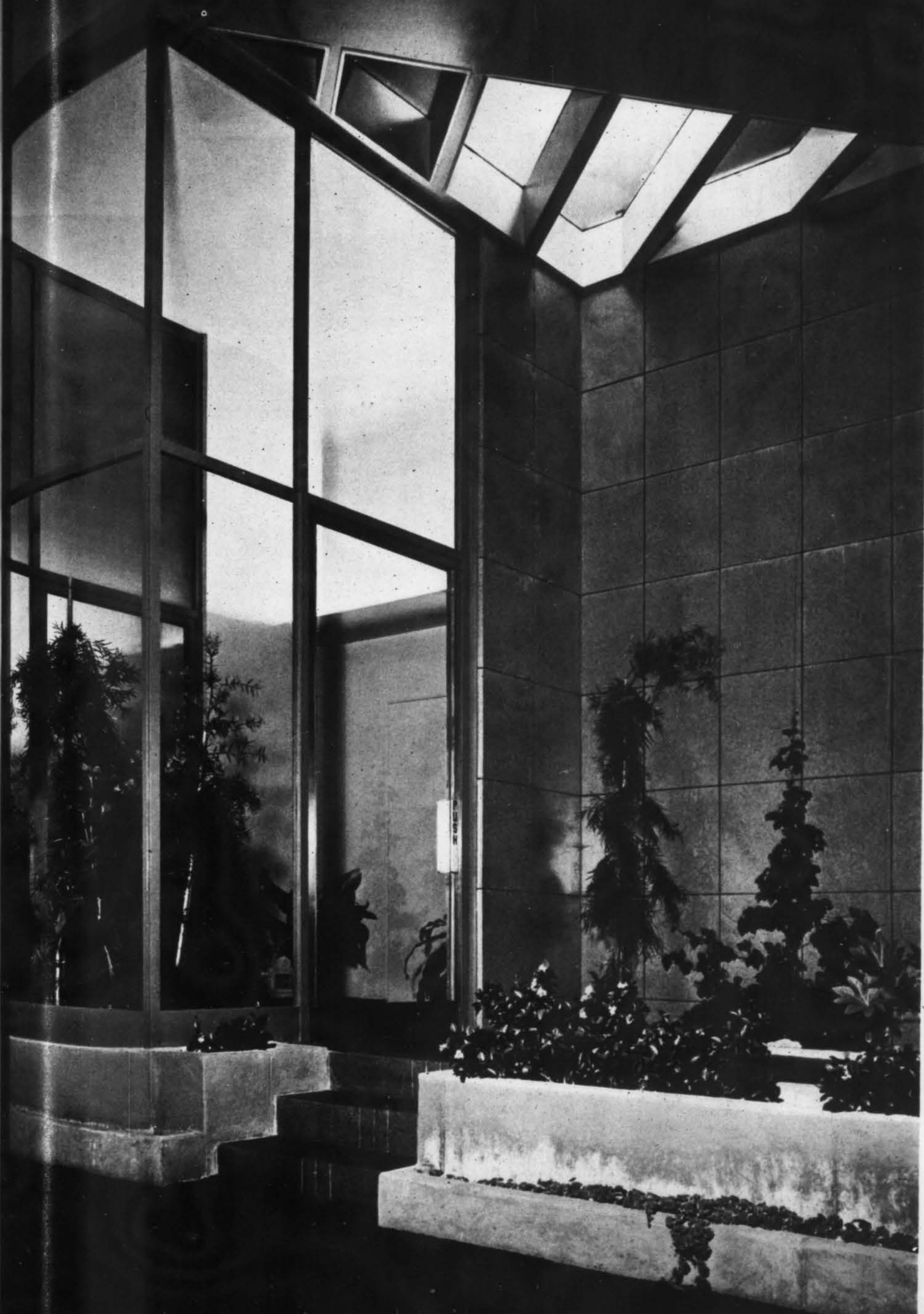
Main entrance and vestibule of the new medical building designed by J. R. Davidson. Glass enclosure with steel frame painted green. Door in stainless steel Exterior wall of ceramic veneer in buff with blue-green overlay and dark brown spots. The floor is dark brown-black terrazzo with design in white metal divider strips.
