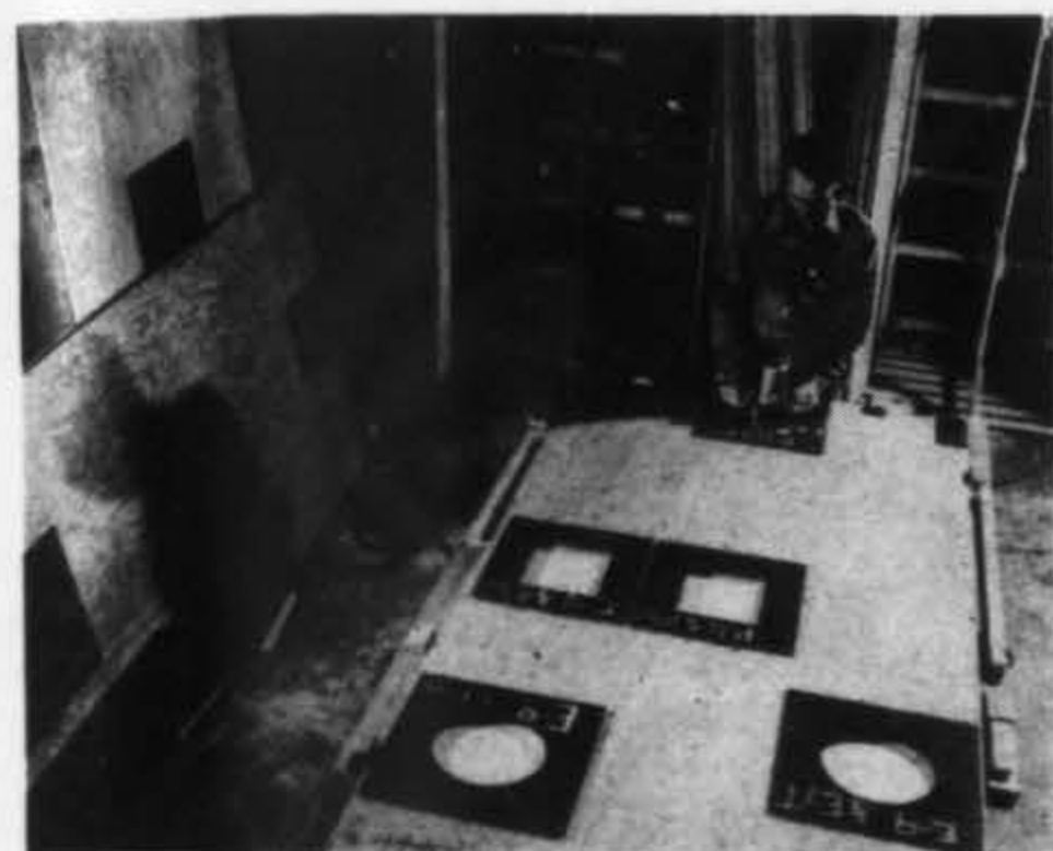
Router operations for utility outlets
