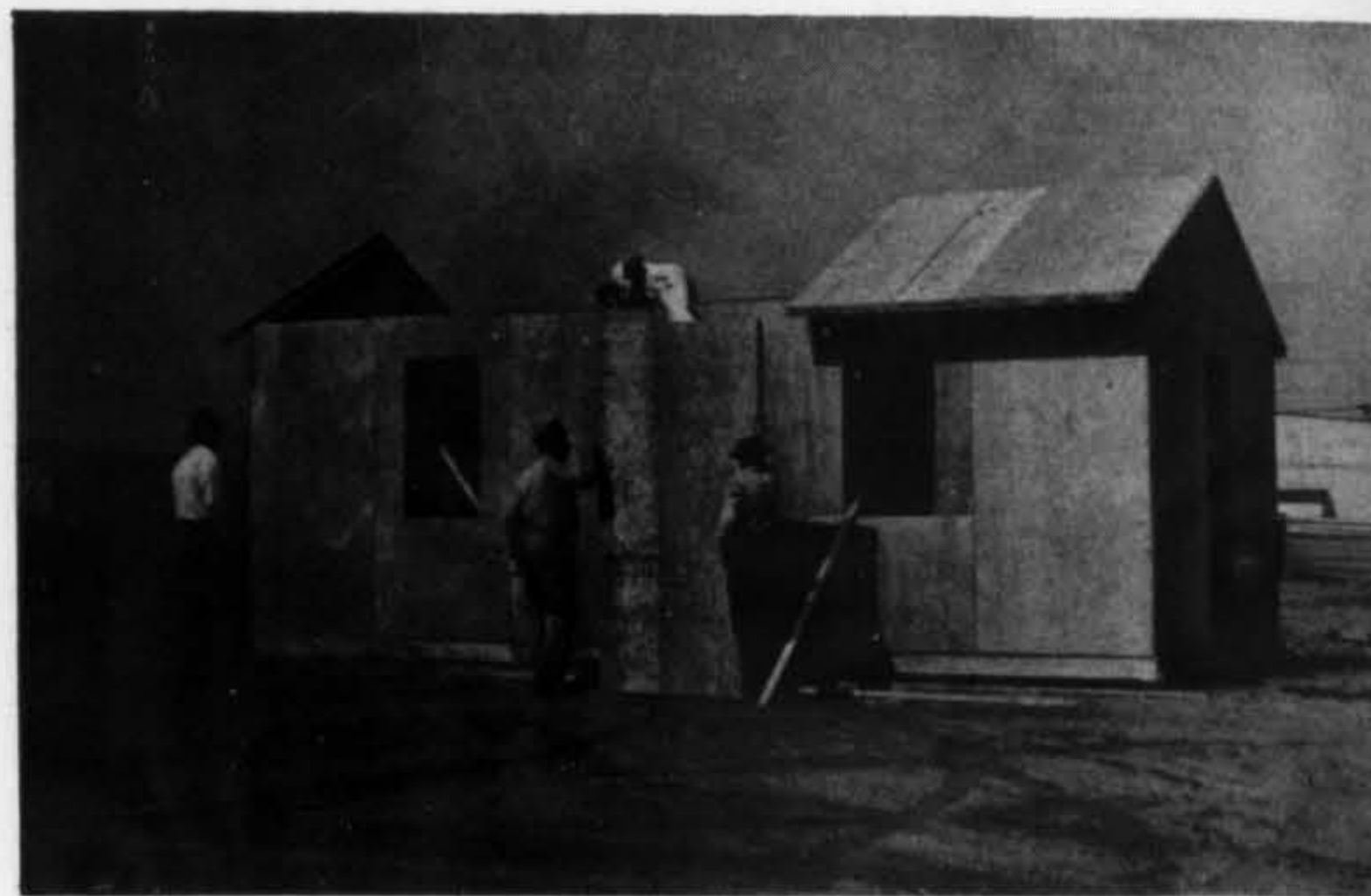
"Prejab" House During Erection
