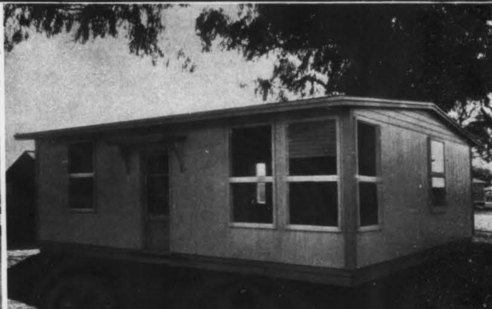
"Victory House" random board prefabrication
