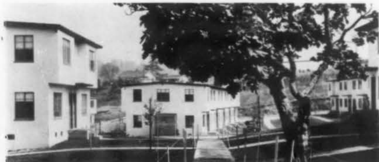
Rose Hill Courts is still another west coast project emphasizing how completely Marlite measures up to the all-out demands of all types of wartime building everywhere.
