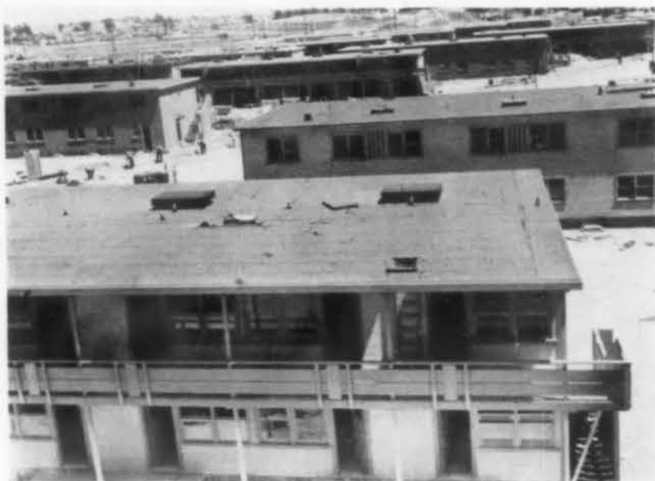
Prefabrication of 1,000 Marlite showers helped speed the completion of the Victory Apartments for 1,000 California war workers and their families at Vallejo.
