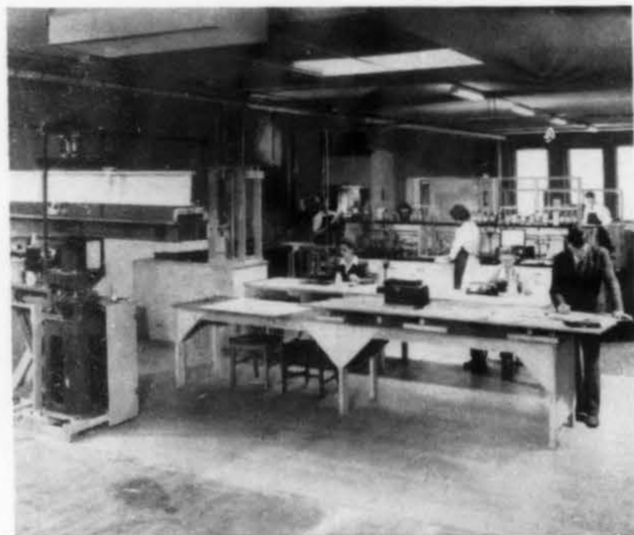
Plywood proving ground. This is a general view of part of the Douglas Fir Plywood Association research laboratory which was expanded under the guidance of Research Chief Arneson. Testing here is designed to increase constantly plywood's performance and develop new uses. Machine in left foreground is for compression tests; other equipment visible includes chemistry bench, weatherometer, drying oven.
