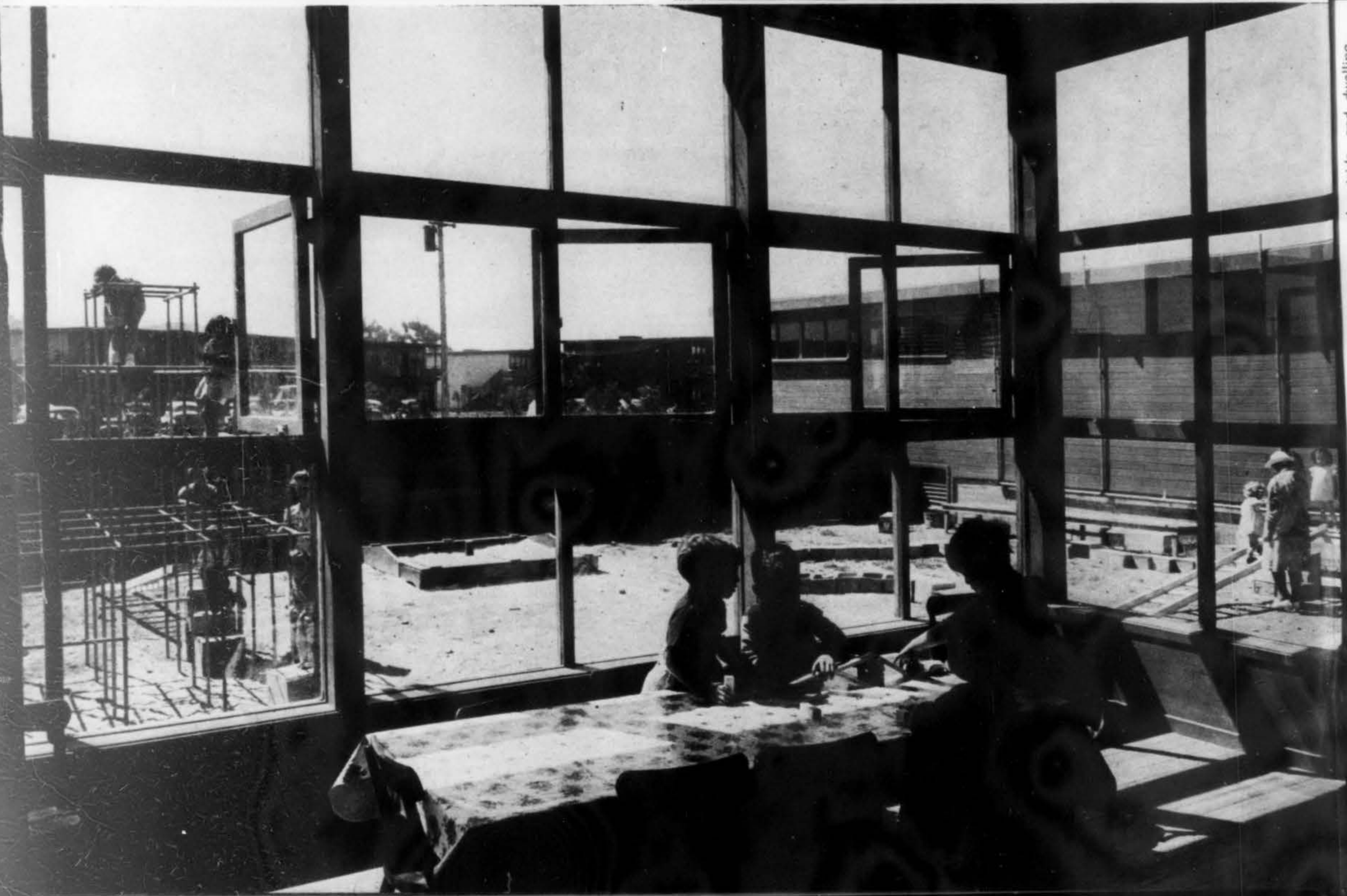
Opposite page (bottom): Interior of day nursery yard, Victory Apartments, nursery yard outside, and dwelling
