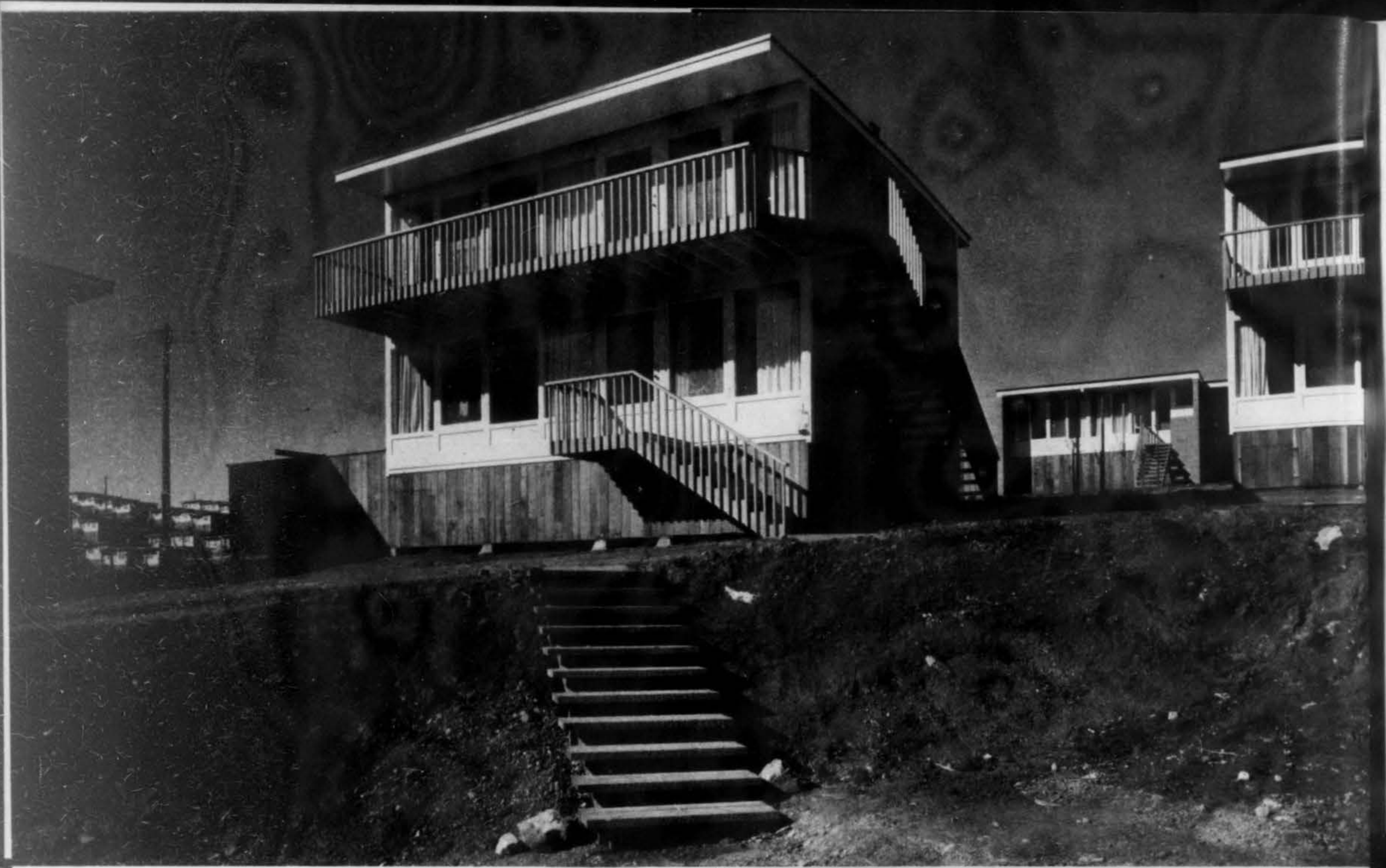
Carquinez Heights experimental units using skeleton frame construction designed by William Wilson Wurster, architect.
