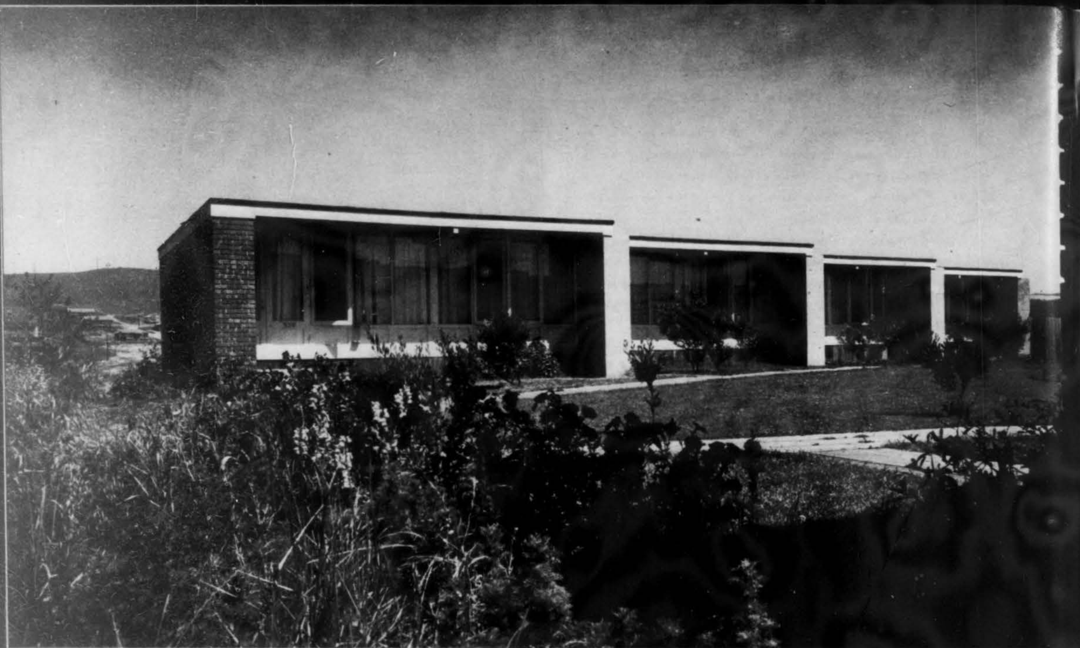
The third type of experimental unit in Carquinez Heights uses masonry wall construction of four kinds of materials for the purpose of comparison.
