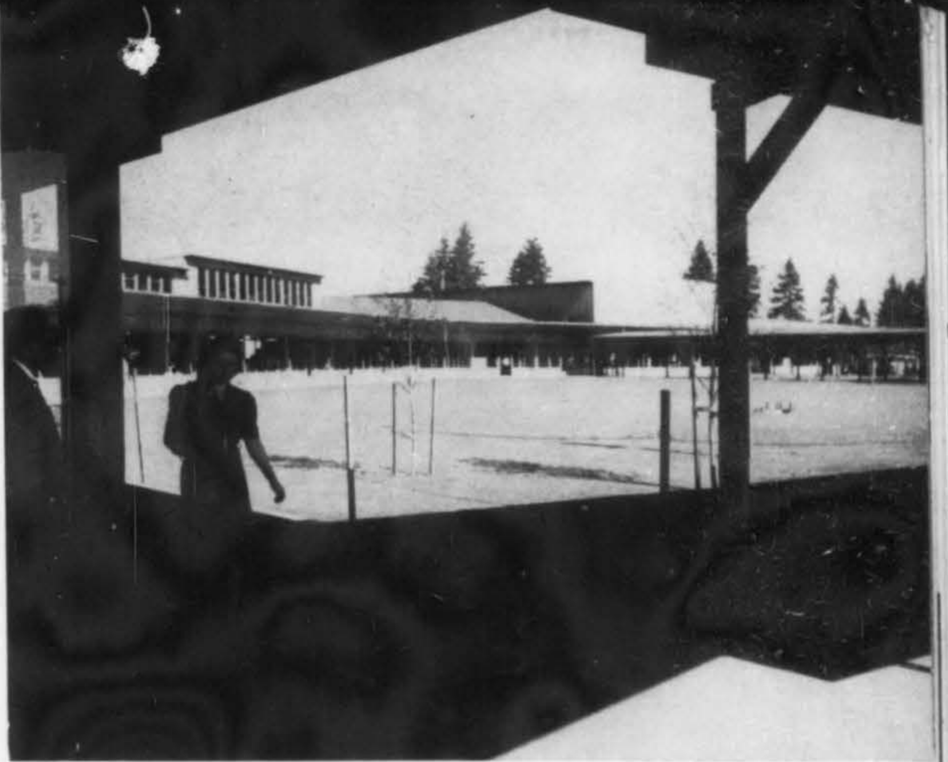
ABOVE: COMMERCIAL CENTER, INCLUDING ESSENTIAL SERVICES & SHOPPING FACILITIES
