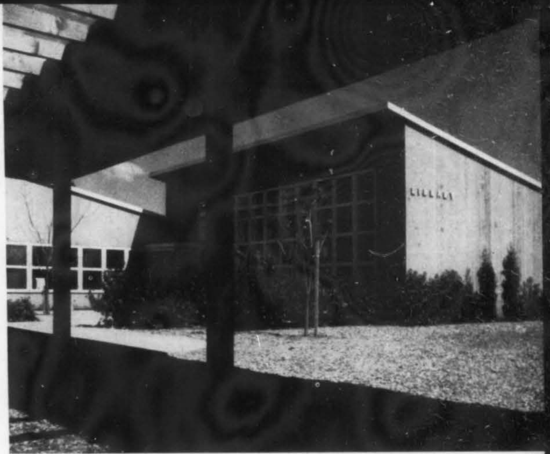
DAY NURSERY IN THE COMMUNITY BUILDING OPENS TO PLAY AREA AND WADING POOL ▲ LIBRARY IN THE COMMUNITY CENTER, OPPOSITE THE GYMNASIUM-AUDITORIUM
