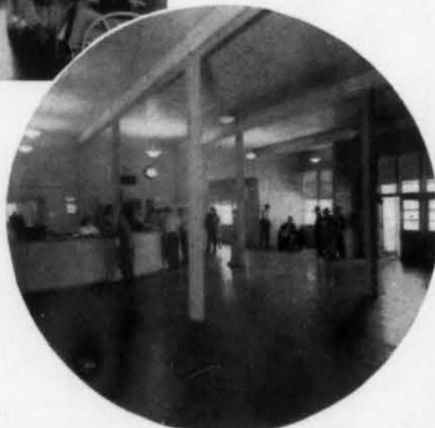
LOUNGE—New technique of applying plasterboard by the use of Laucks Construction Glue in place of nails, speeded the installation of these lounge walls, saved steel, and eliminated defacing nail holes.
