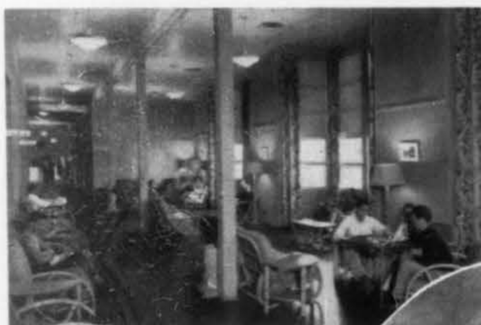
LOUNGE—New technique of applying plasterboard by the use of Laucks Construction Glue in place of nails, speeded the installation of these lounge walls, saved steel, and eliminated defacing nail holes.
