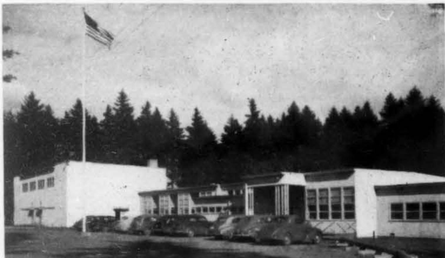
ADMINISTRATION BUILDING—Rezitex . . . synthetic resin, plastic-type paint . . . on exterior grade fir plywood gives this beautiful Ogden Meadows administration building its appearance of monolithic concrete.
