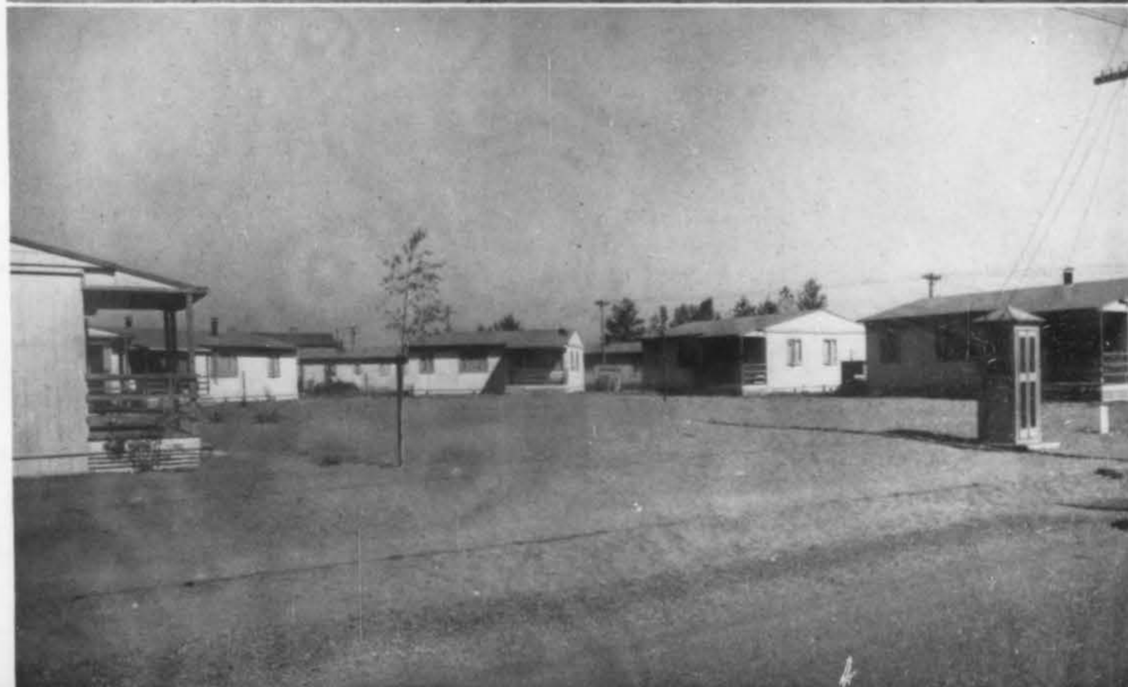
FROM TOP TO BOTTOM: A SMALLER ADMINISTRATION BUILDING AT HUDSON STREET HOMES; FULTON COURT; PARKSIDE HOMES.
