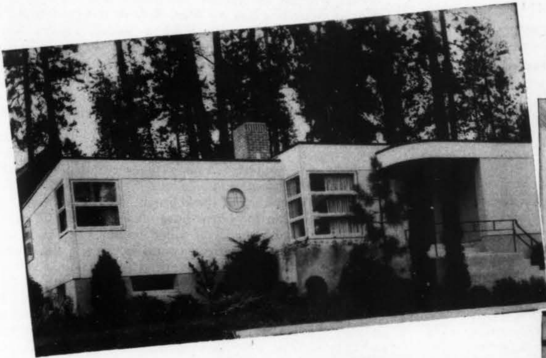
Design of this attractive, durable home relied upon smooth exterior walls of plywood for appearance value. Edwin J. Peterson, architect.
