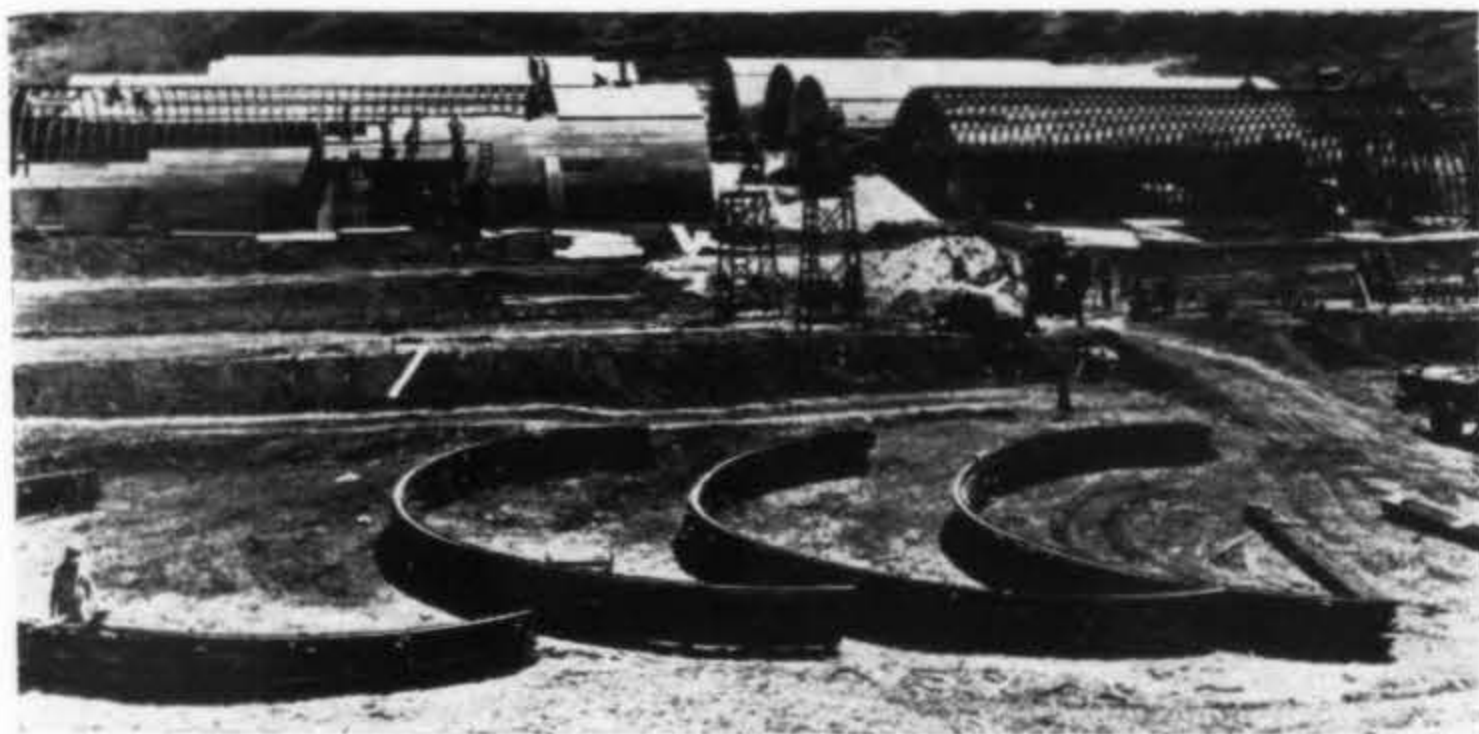
Stran Steel arches ready for use for warehouses in the South Pacific. Note building ready for covering. Official U. S. Navy Photograph.
