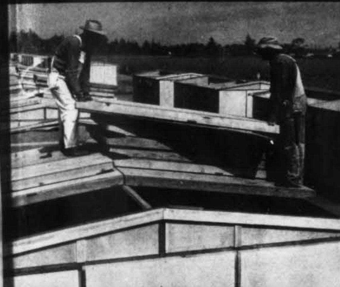
ON GOES THE ROOF
