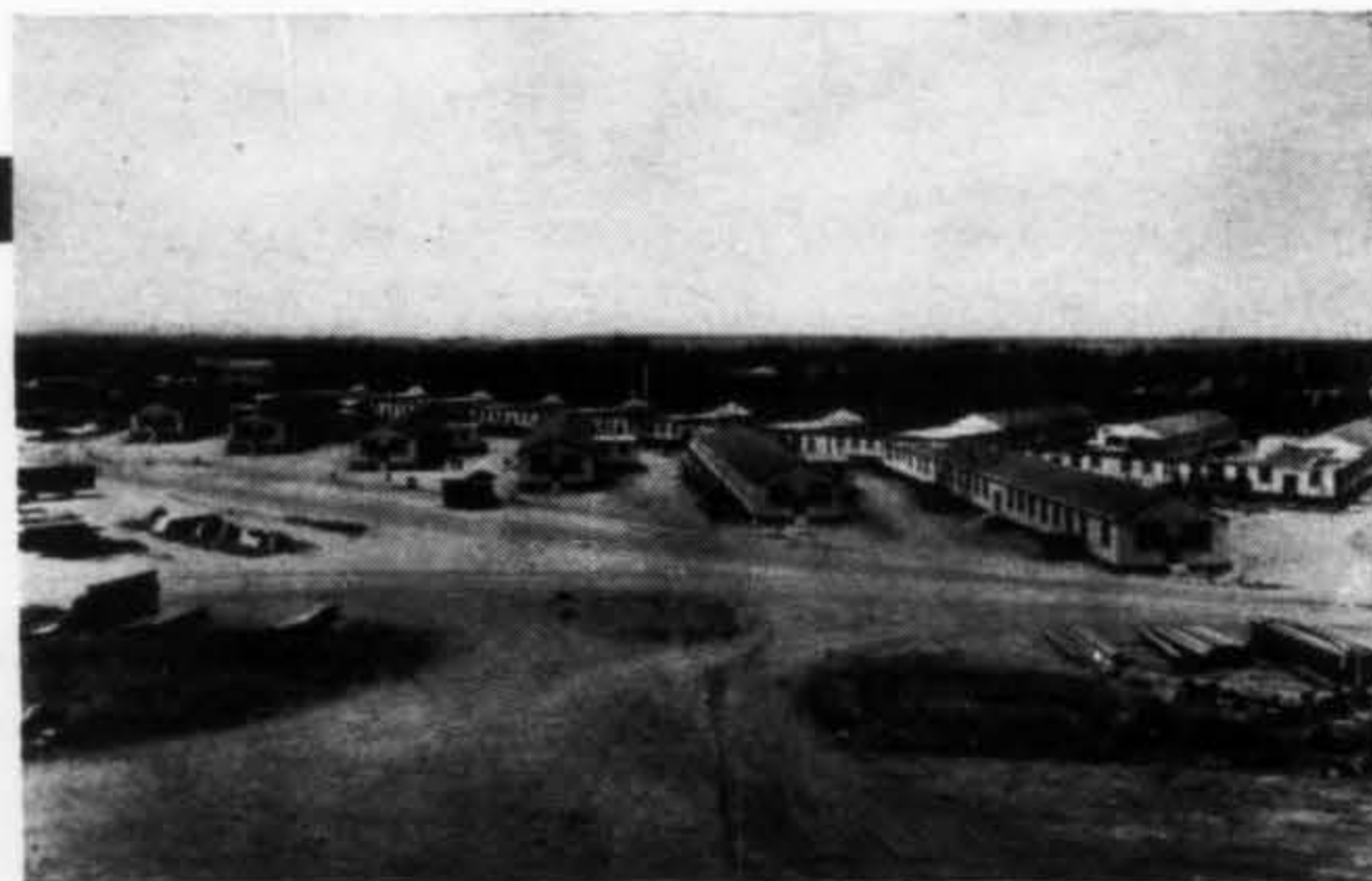
Panorama view of part of Naval Hospital at Corona, California, built with Modulok Cemesto Wall Units.
