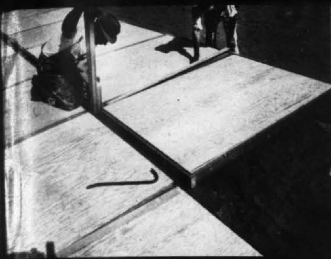
FLOOR PANELS FIRST
