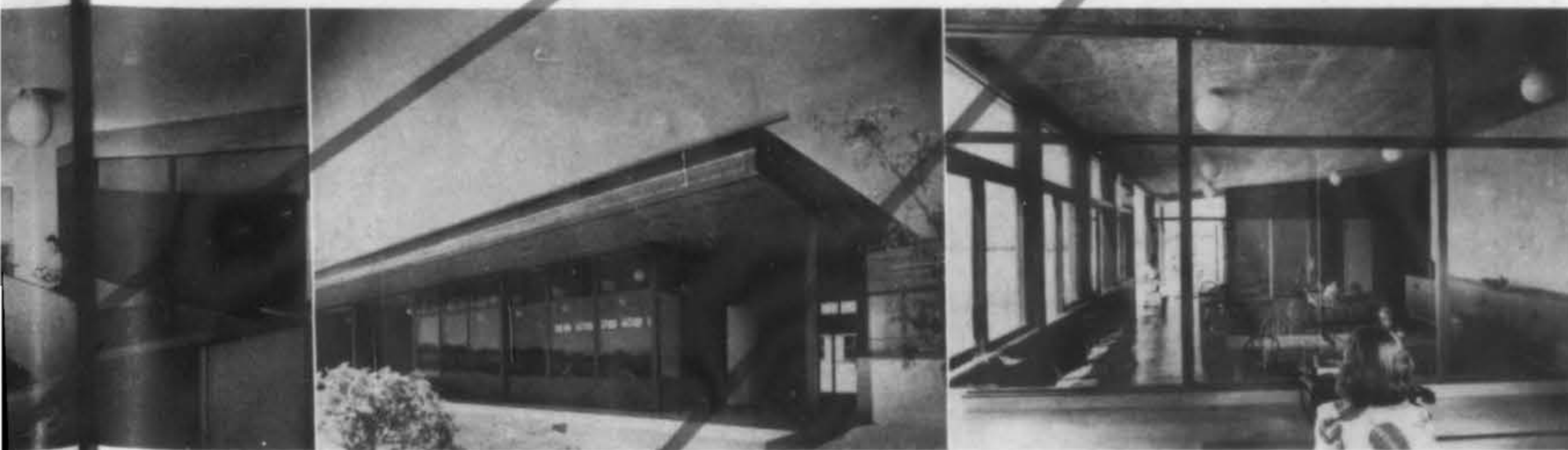
Above: the Community Center arcade leads to the nursery school. Center: Assembly Room wing of Community Center. Right: Nursery School Play room is easily policed.
