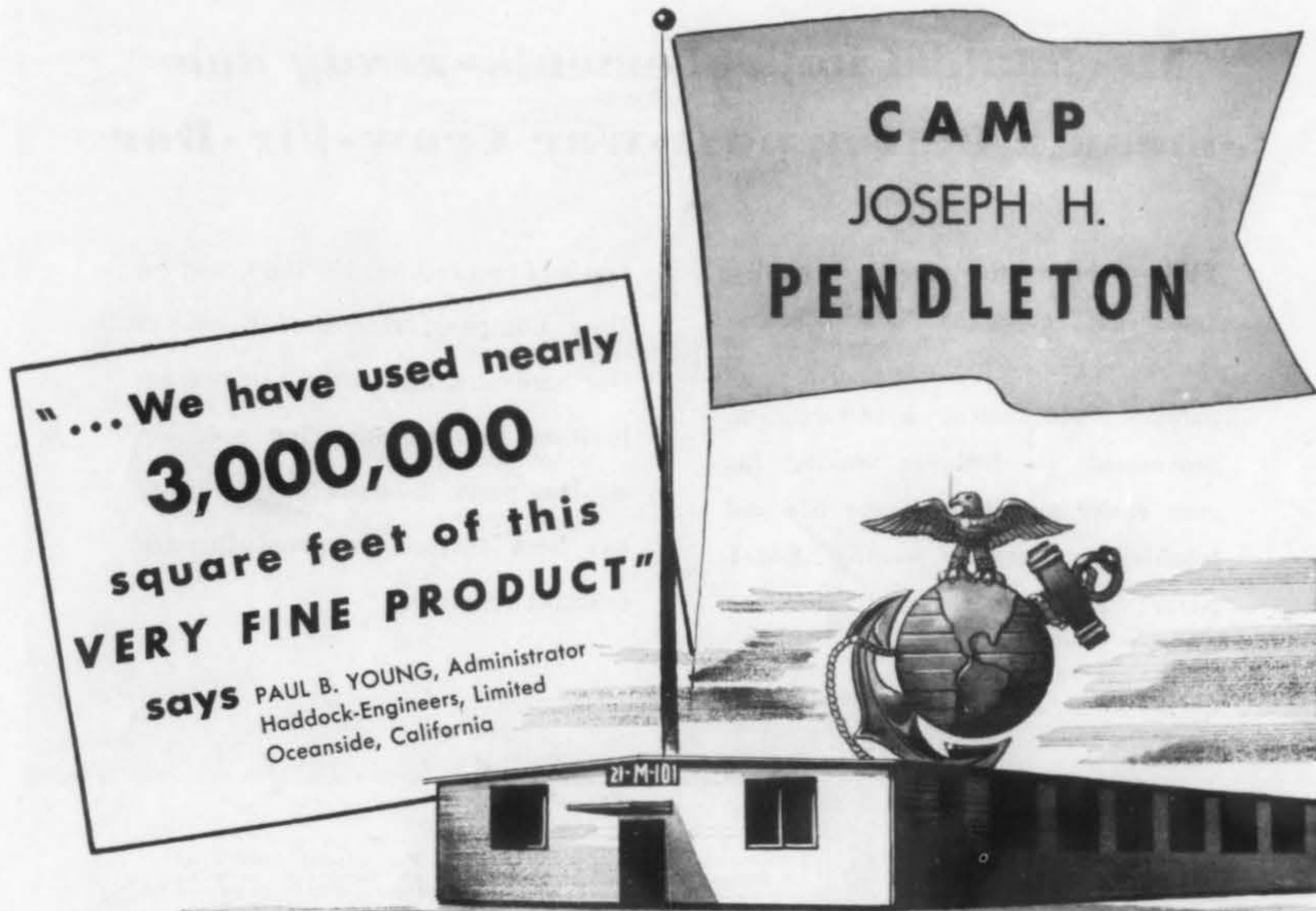
One among the hundreds of buildings constructed at Camp Joseph H. Pendleton.
