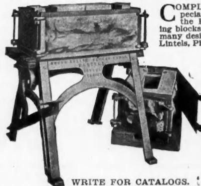
COMPLETE in every detail. Especially adapted to the use of the Block manufacturer. Making blocks in all widths, lengths and many designs, including Sills, Lintels, Pier Blocks etc. PRICE \$100
