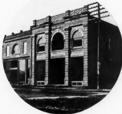
two-piece building blocks of the wet mixture, 1 to 2 to 3. This building is 37 by 60 feet and was erected last fall at a cost of \$5,600. All the molds and forms were made by myself and this building has proved to be warm and dry during the past winter and is admired by all. CHAS. L. SCOTT.
