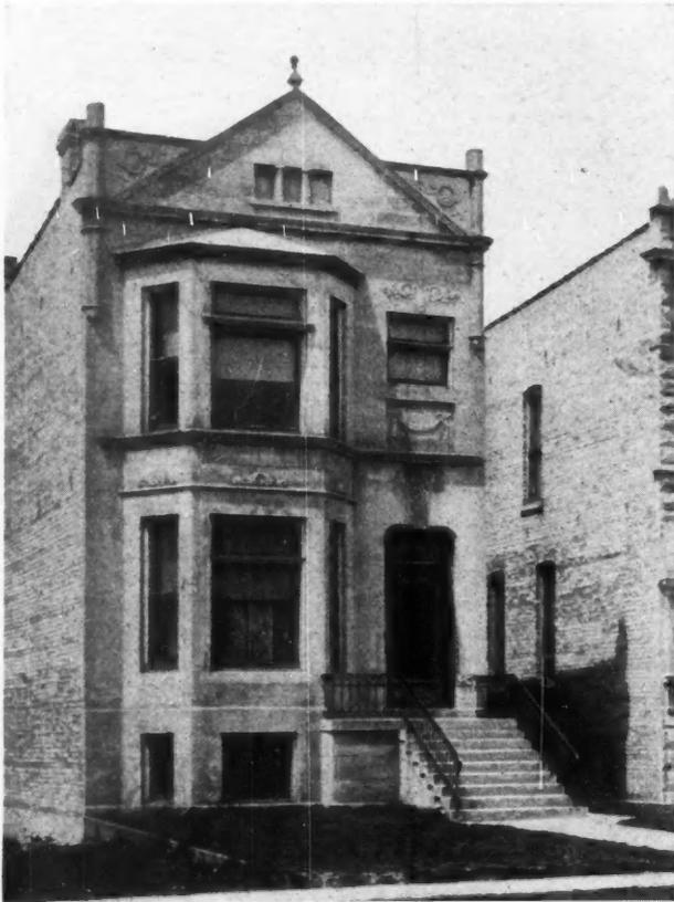
Well-Planned 2-Flat Building—Brick with Cut Stone Front
