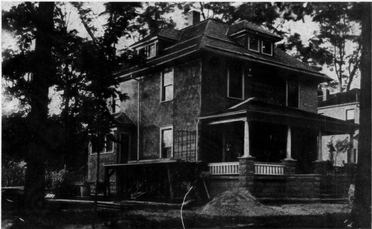
**House at Niles with "Scratch" Coat Partially on. Note Furring Strips and Lath**
