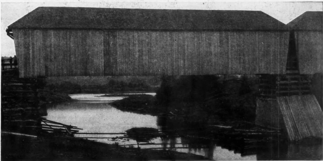
Fig. 3. Modern Wooden Bridge, Covered to Protect the Timbers
