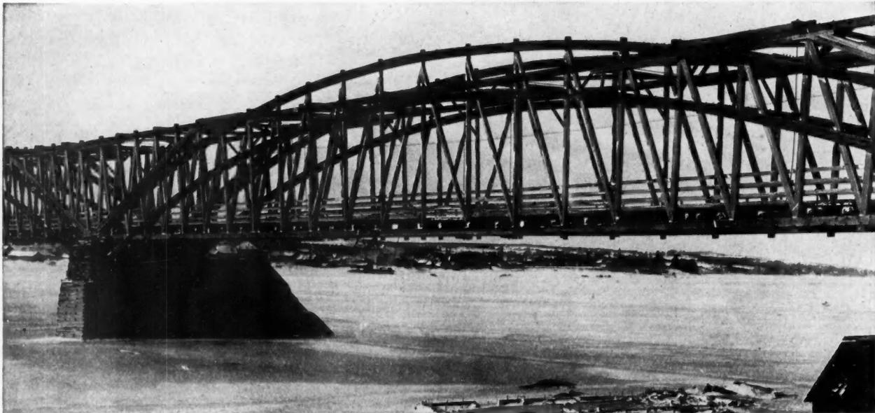
Fig. 1. A Fine Old Wood Truss—240 Foot Span
