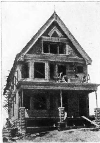
as to the angle at which it rests to the building, so shifting the weight that a thousand pounds is easily carried at the extreme outward end of the bracket, making a scaffold as safe for the carpenter to work on as though he were upon the ground.
