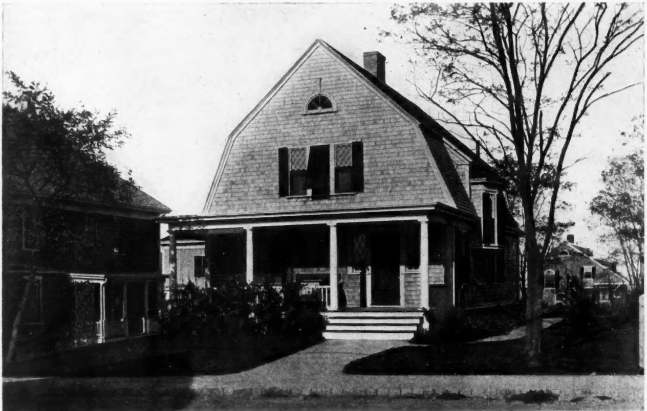
[Gambrel]Roof House with Shingled Walls Built at Plymouth, Mass., for \$3000; W. F. Barlow, Jr., Brockton, Mass., Architect
