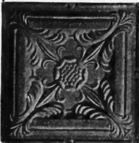
Quickly and easily applied. We are the only manufacturers who cut the heads in the dies after casting. Result—Square and accurate plates—which will save you time and labor in cost of erection.
