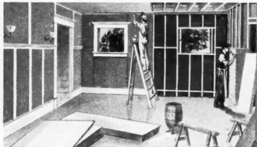
*Nailing Beaver Board to the Walls and Ceiling of a New Room.*
