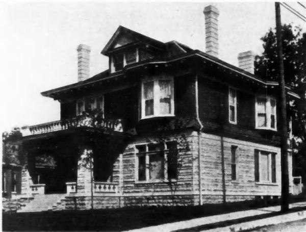
Rough Finished Blocks in Two Widths in Combination with Shingles
