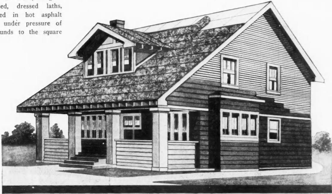
Bishopric Sheathing Used Under Clapboards and on the Roof Under Ready Roofing
