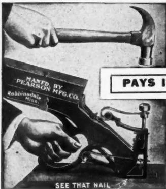
Works well on any pitch roof. Gloves or mittens can be worn and nails driven faster than by the old way. Throw nails in by the handful—holds about 600 nails—start nailing. Nails can be driven through tin or quite heavy sheet iron.
