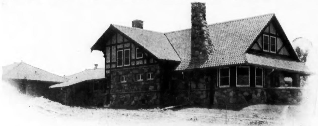
Striking Work With Field Stone on Residence of Mr. M. Ford, at Cedar Rapids. Chimney, Laid up by Frank Klepach, is especially good
