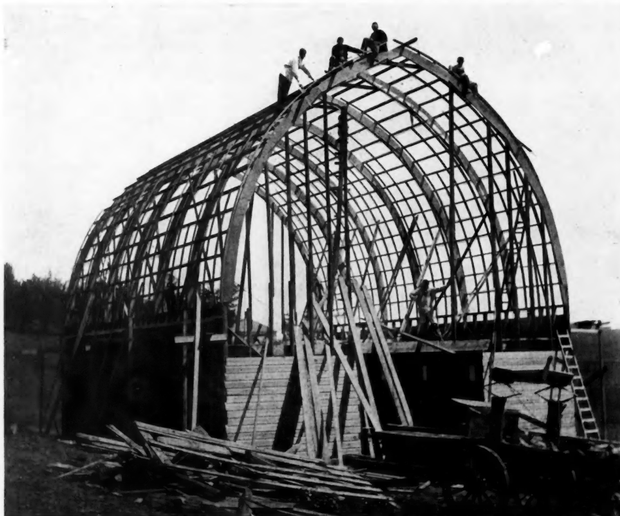
WM. STEINER AND MEN FRAMING GOTHIC ROOF BARN AT JOHNSON, WASH. Curved Rafters are Sawed Out 1 by 12's and Nailed four together.
