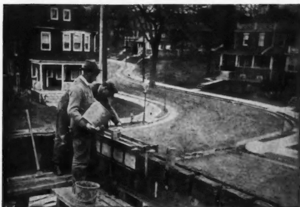
Making ready to insert the floor beams.
