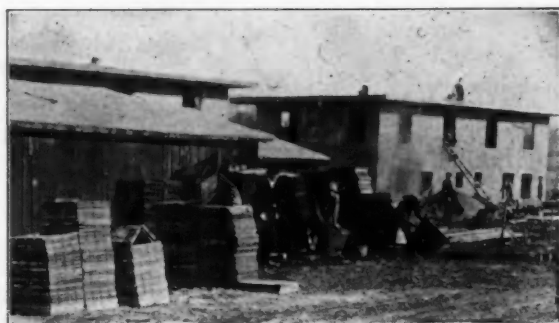
Morrill Steel Forms Used on the "Concrete City" at Nanticoke, Pa., for the D. L. & W. R. R. Co.
