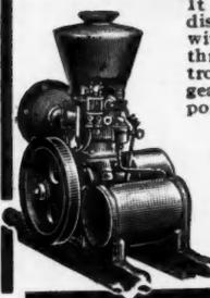
It runs on kerosene (coal oil), gasoline, alcohol or distillate without change of equipment—starts without cranking—runs in either direction—throttle governed—hopper cooled—speed controlled while running—no cams—no valves—no gears—no sprockets—only three moving parts—portable—light weight—great power—starts easily at 40 degrees below zero—complete, ready to run—children operate them—5-year ironclad guarantee—15-day money-back trial. Sizes 2 to 20 horsepower.
