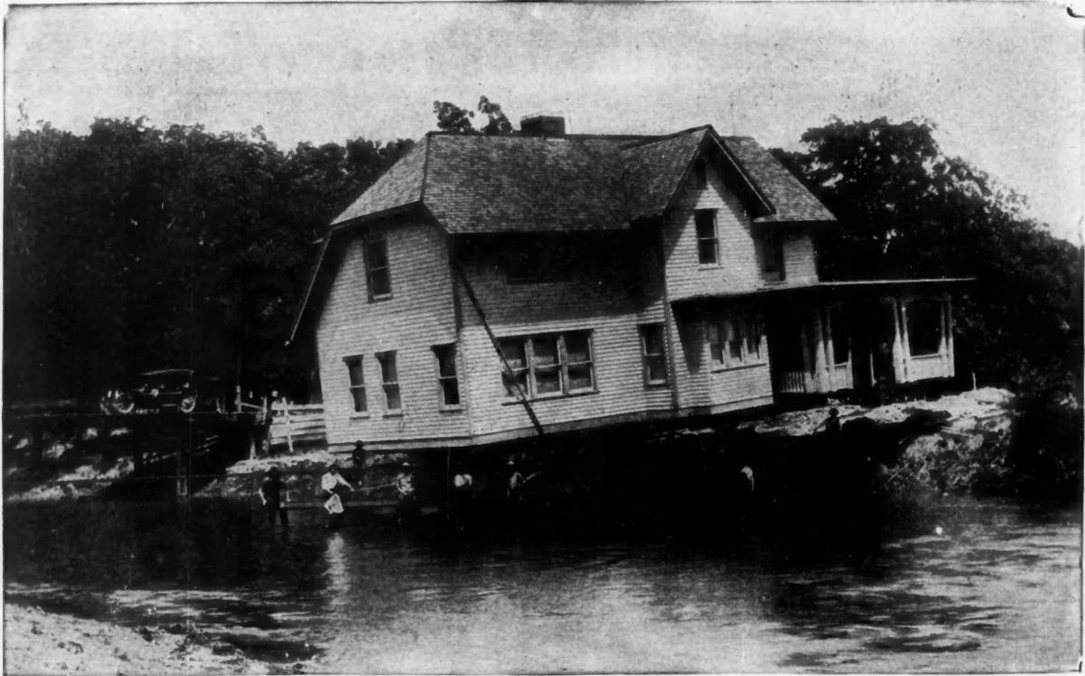
Ten-Room House Moved Across the River by R. C. Cole, Moline, Ill., Without Cracking Plastering or Paper
