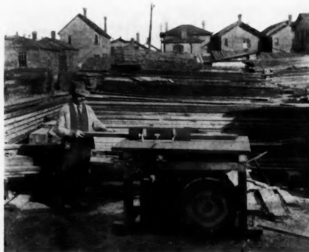
"Wonder" Saw Rig Working up Form Lumber.
