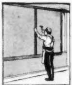
Decorative strips are nailed over edges after painting.
