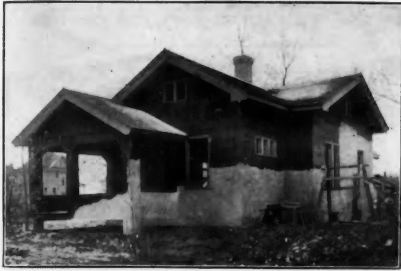
RIB LATH Residence of H. A. Ertz, St. Paul, Minn., during construction.
