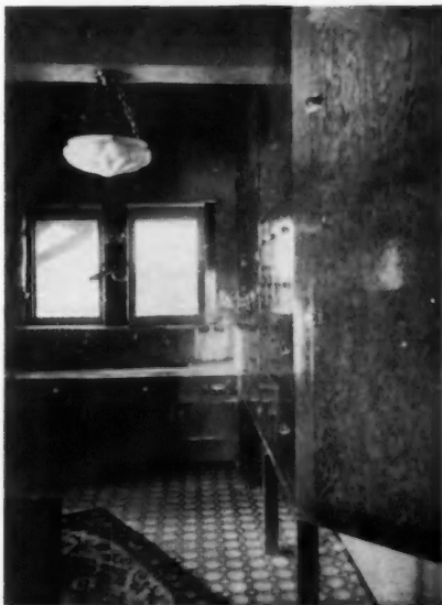
Kitchen. On the right the built-in Cupboards, Refrigerator, Bins, etc., with Sliding Tables beneath; water heater on extreme left over Sink; Washing and Drying Appliance in center of wall; Garbage Chute in lower right corner.
