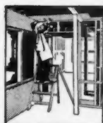
Method of support- ing ceiling panels
