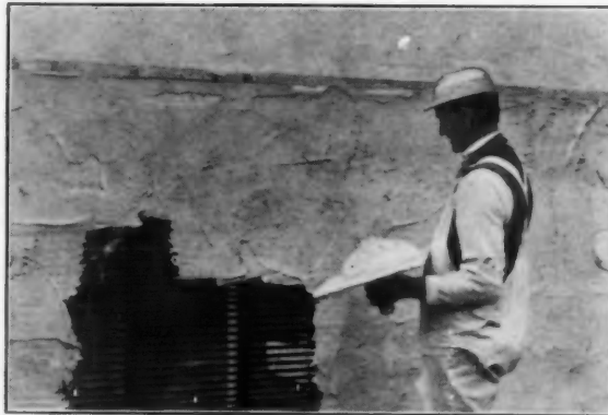
Note perfect clinch of plaster on RIB LATH, with no dropping off.
