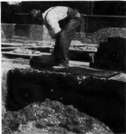
On top of the concrete foundation the men laid a damp proofing course of asphalt soaked paper to keep moisture from creeping up.
