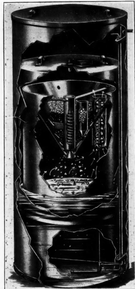
Interior mechanism of "Faultless Pit" Acetylene Generator.
