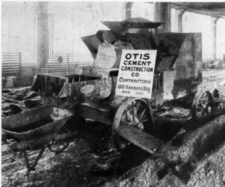
A Double Trough "Hartwick" Continuous Mixer Laying 150,000 Square Feet of Concrete Floor in the Detroit-Paige Motor Company's New Factory, Detroit, Mich. The Otis Cement Construction Company, Contractors. This Machine has been in Hard, Continuous Service for Seven Years.
