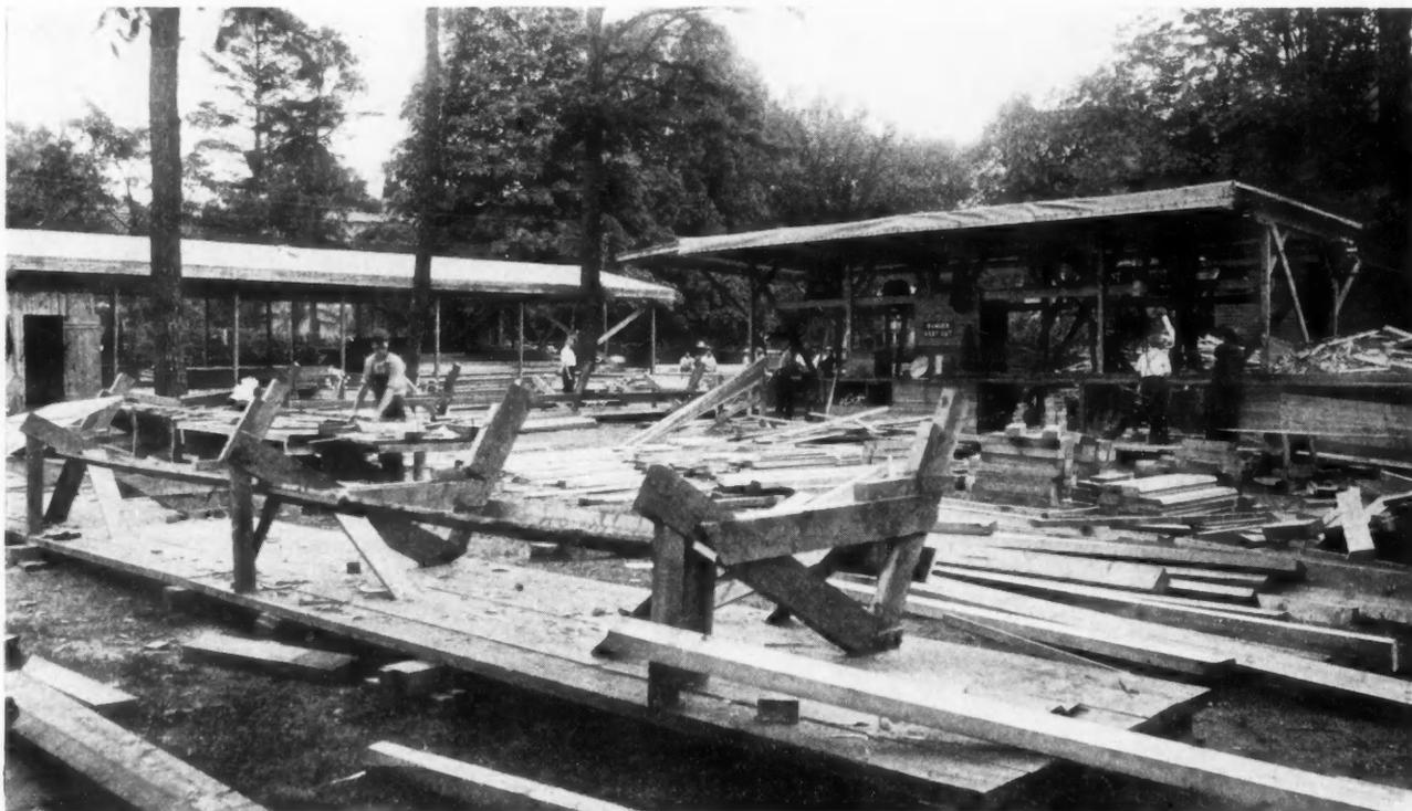
Photograph of Carpenter Shop With Power Equipment as Used by the Aberthaw Construction Co. of Boston, for Making Wood Forms for Large Reinforced Concrete Jobs. This is the Arrangement of Saw Mill, Lumber Piles, and Erecting Horses They Have Found Most Economical and Have Made Standard on Their Work.
