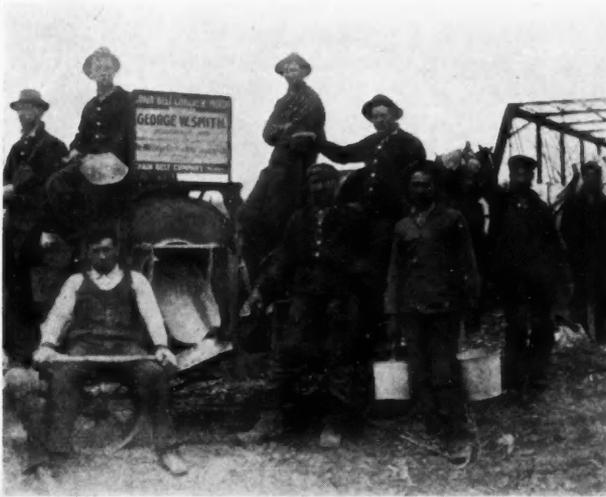
Bridge Work is Profitable When Done with a Power Mixer. Contractor Geo. W. Smith, of Belleville, Ohio, and His Crew Discovered After Just Finishing a County Road Bridge with the Help of a "Chain Belt" Mixer that Averaged 100 Cubic Yards of Mixed Concrete Per Day.
