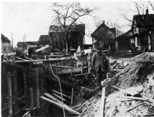
No Lost Motion on this Foundation Job. The "Crescent" Continuous Mixer is Placed Right Up to the Trench and Deposits Directly into the Forms. Clean Sandy Gravel was Excavated from the Building Site so that Here No Hauling of Material was Necessary, Either Before or After Mixing.
