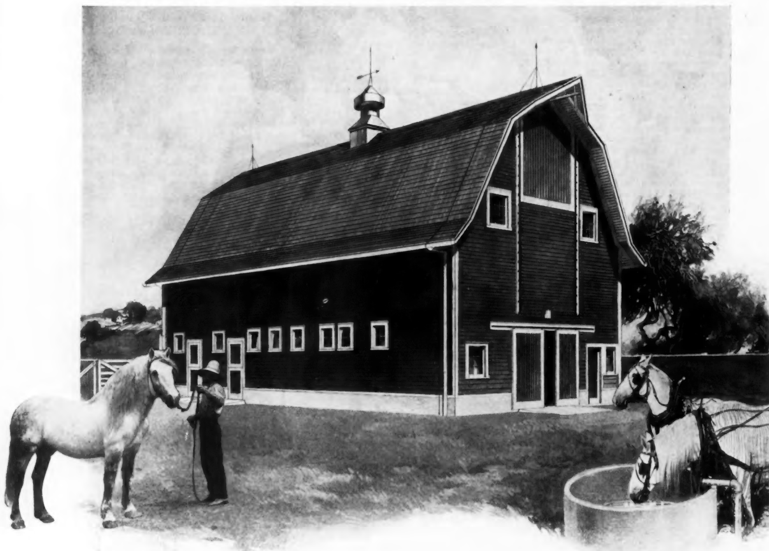
Horse Barn Design Measuring 66 by 32 Feet, 20 Feet High to Plates, with Full Self-Supporting Gambrel Roof. A Modern Horse Barn in Every Particular. Any inquiries in regard to equipment or plans for this Horse Barn will be given prompt attention.—Editor.
