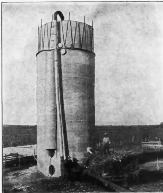
Poured Concrete Silo with Metal Roof Extension for Silo Filling. With this Type of Roof Our Silos are Brimming Full, Even After the Silage Has Settled.
