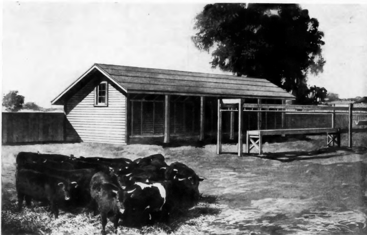
Design for Stock Feeding Shed Opening Toward the East. This Shed Measures 52 by 16 Feet. It is Constructed of 2 by 4 Studs Set in Wrought Iron Studding Sockets on Solid Concrete Footings. Trolley Track Feed Carrier Service Brings Silage and Other Feed to Open Feed Racks.
