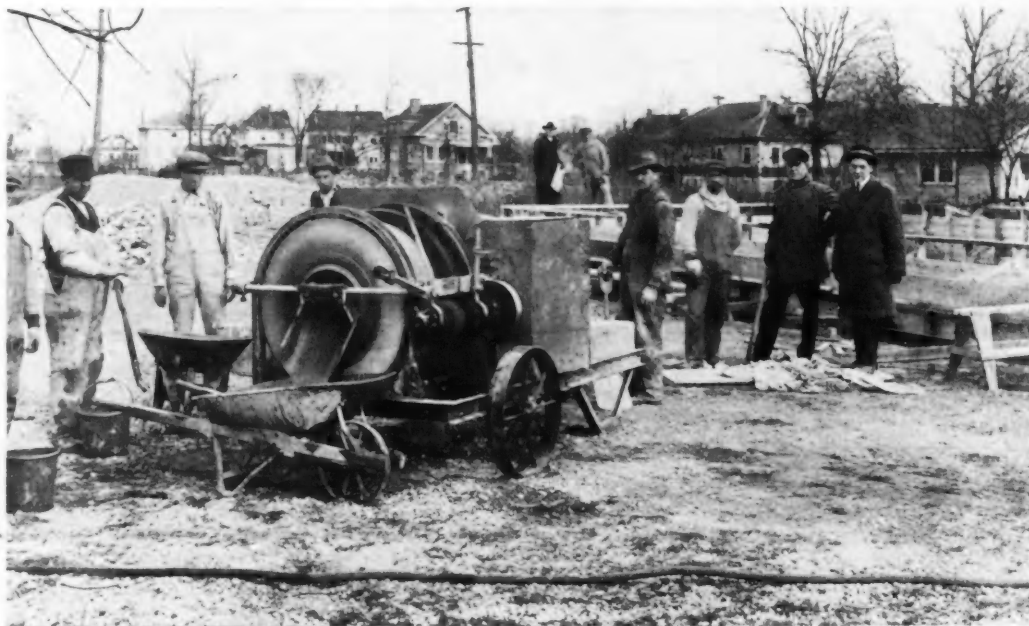
"Little Devil" Mixer on Two Wheels, with Charging Spout and Holst.
