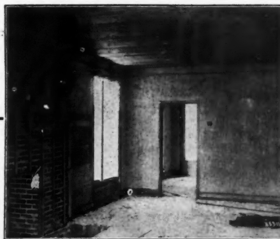
Rib Lath as Used for Partitions, Ceilings and Furring in Detroit Residence.
