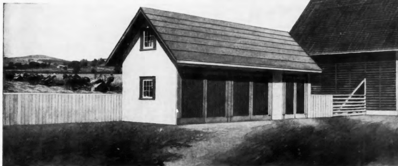
Design for Implement Shed and Farm Blacksmith Shop. Dimensions 48 by 16 Feet. Walls are Constructed of Cement Plaster on Metal Lath, Attached to 2 by 4 Studs, Door Posts, 8 by 8.
