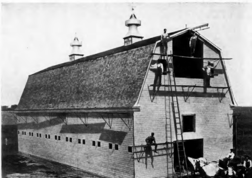
Reliable Scaffold Brackets in Use by Barn Builder John Willmann, Oriska, N. Dak.
