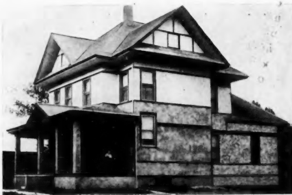
Old Frame Houses are Ideally Remodeled by Overcoating with Cement Plaster on Metal Lath. N. W. Ex. Metal Co.'s "Kno-Burn" Lath was nailed Direct to old clapboards of this house at Virginia, Ill.
