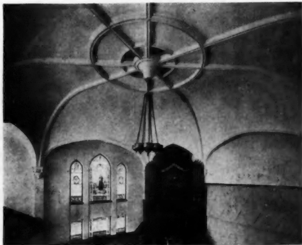
Ceiling of Trinity Reformed Church, Philadelphia. Carl P. Berger, Arch. Lathed with Bostwick "Truss Loop."
