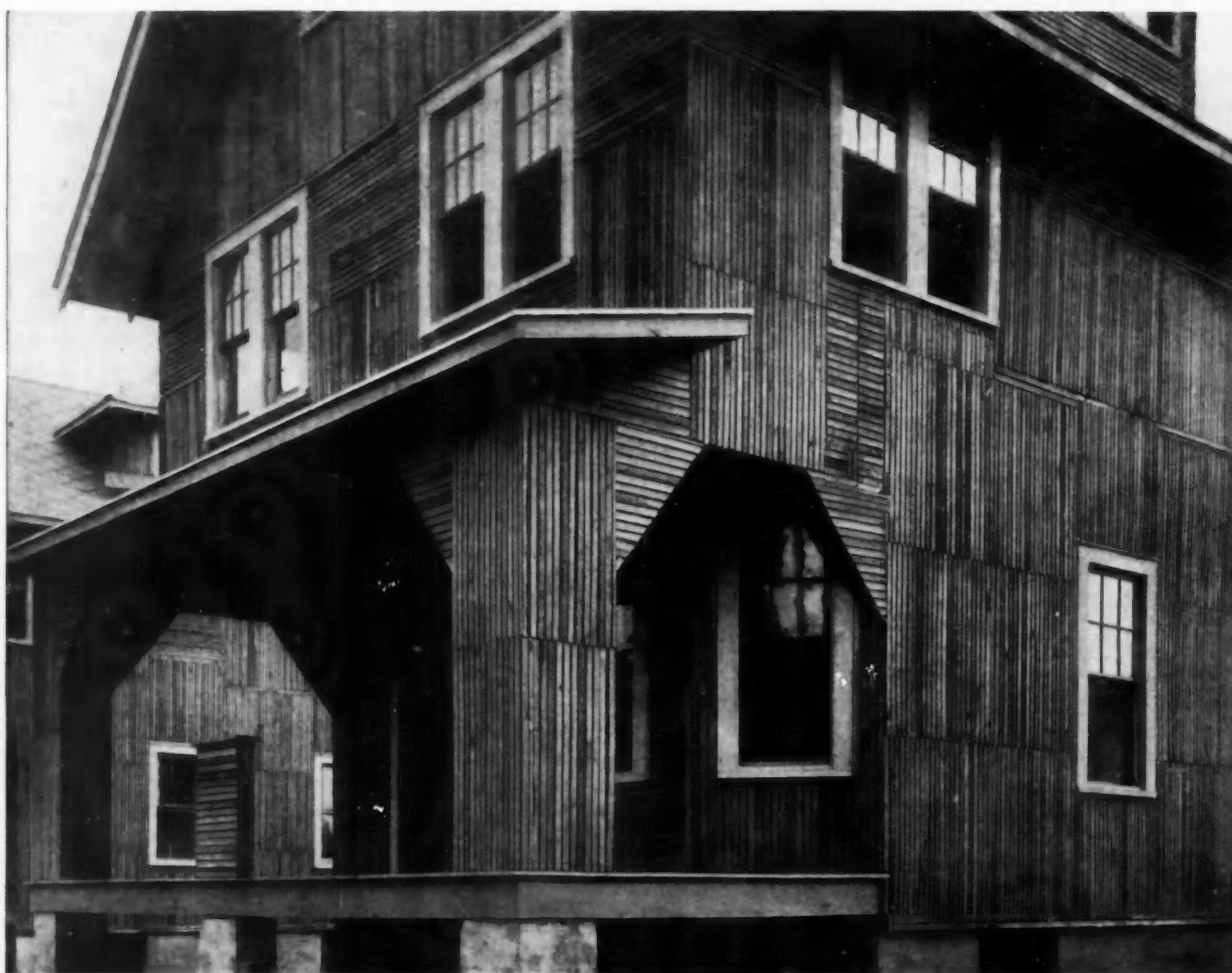
How "Bishopric" Stucco Board Looks on the Wall—All Ready for Cement Plastering. Photo of a Group of Fine Residences Being Put Up by the Passaic Building Co.
