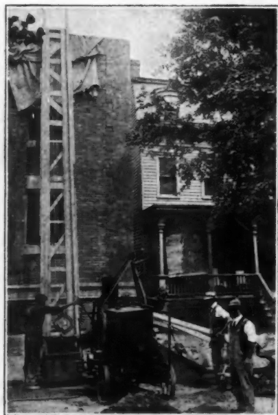
Mixer with Hoisting Attachment.
