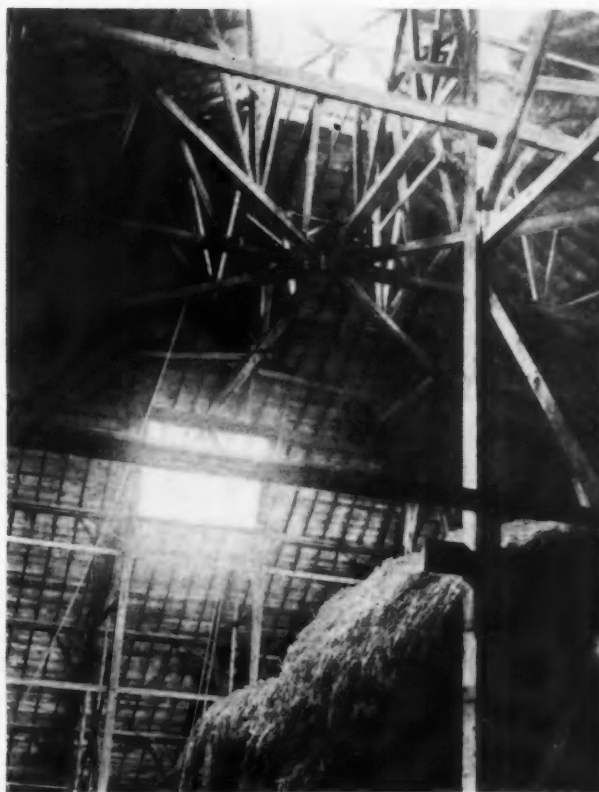
Interior Photo Showing Framing Underneath the Cupola.
