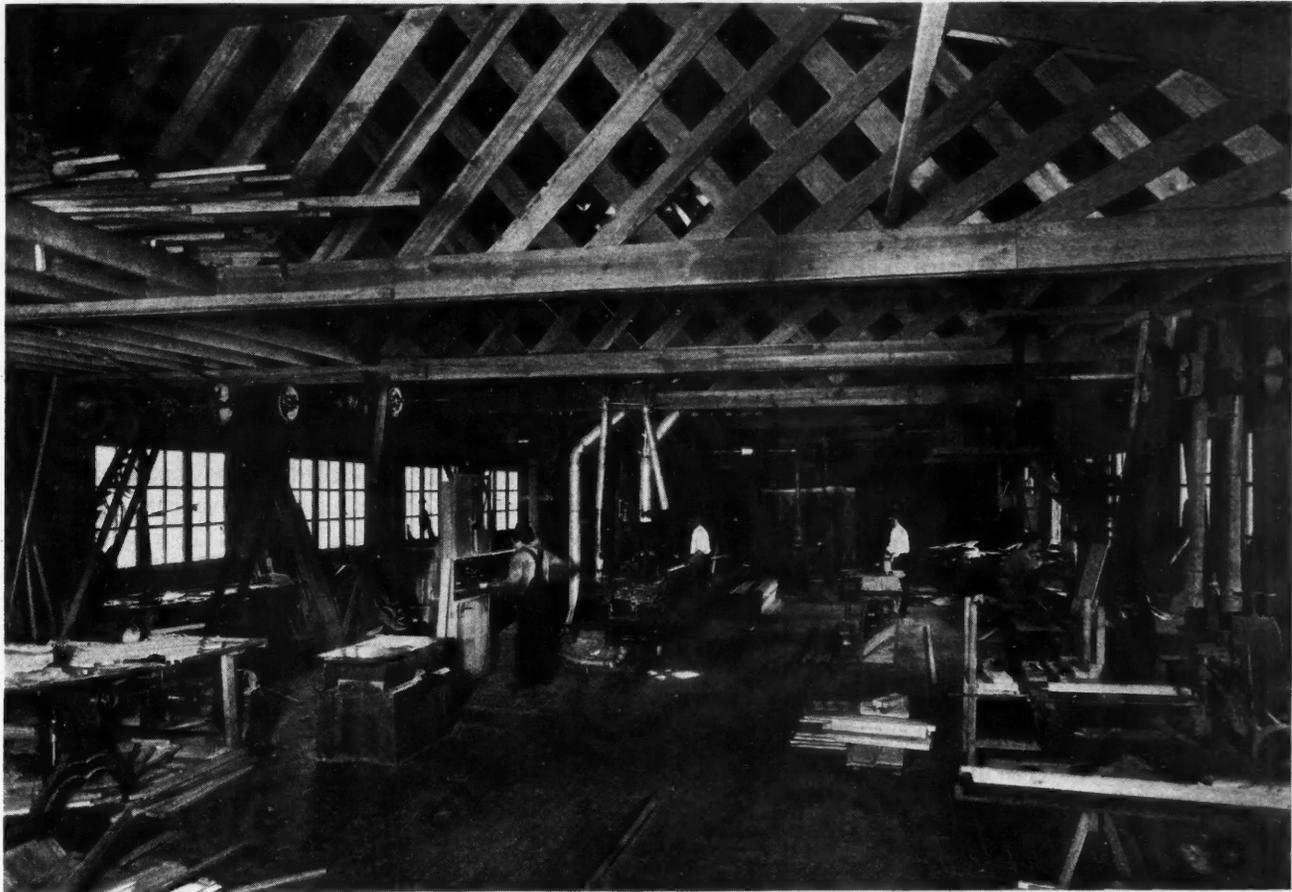
Interior View of the Wiederhold Lumber & Mfg. Company Shop. Blower Exhaust System Carries Away All Sawdust and Shavings to Outside Fireproof Bin of Hollow Tile Construction.
