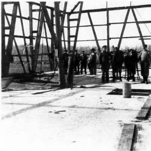
Concrete Floor as Placed Over First Floor and Under Hay Mow.
