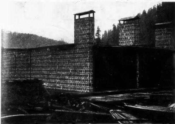
Hollow Tile Dry Kiln of the Mineral Lake Lumber Co., Mineral, Wash.
