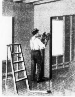
How "Rock-Board" is Nailed to the Studding. Only One Man is Necessary.
