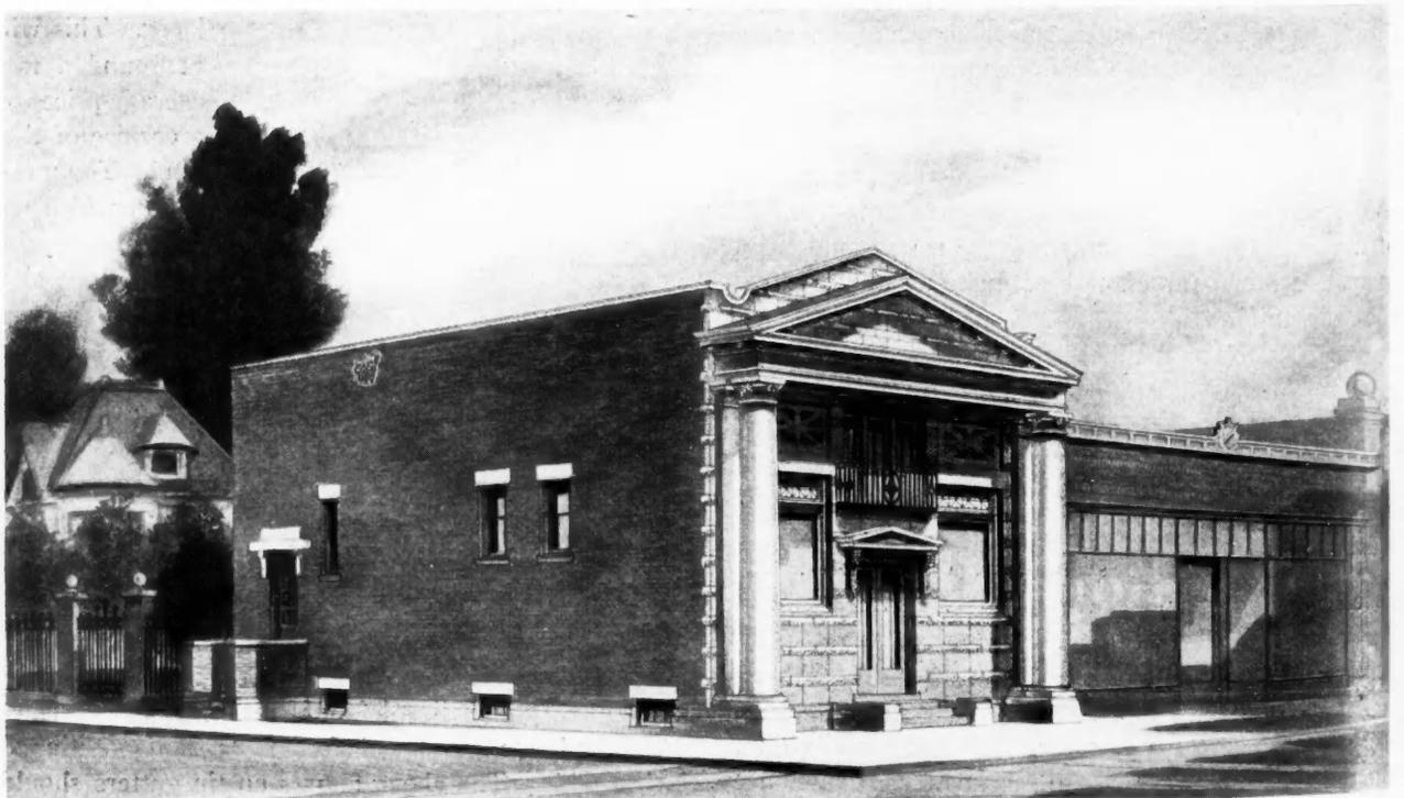
Perspective Sketch of Very Attractive Small Bank Building, Constructed of Brick and Terra Cotta. Dimensions, 25 by 54 Feet. When Writing About This Design Please Refer to Design No. 6748. Price of Blueprints and Specifications on Application.
