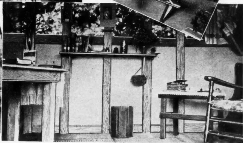
Four Views of Interior of Wall Board Camp Pictured Above. Waterproofed Wall Board Nailed to Rather Heavy Battens Forms All Walls and Partitions. The Roof is Made of Composition Roll Roofing Laid Over Matched Boards.
