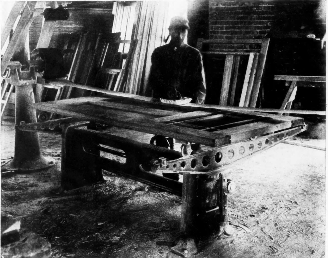
Finishing Stiles and Rails of a Door with the Yates Flexible Belt Sander.
