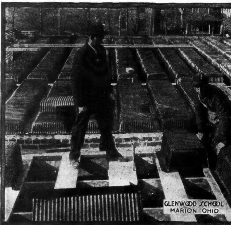
**B**ERGER'S Pressed Steel Cores, for both light and heavy long-span construction, are extensively and effectively used for concrete floors. They are designed to give the greatest strength and displacement for the least amount of weight and cost, at the same time making a great saving in concrete reinforcing steel, centering and labor—also materially reducing the dead floor load.
