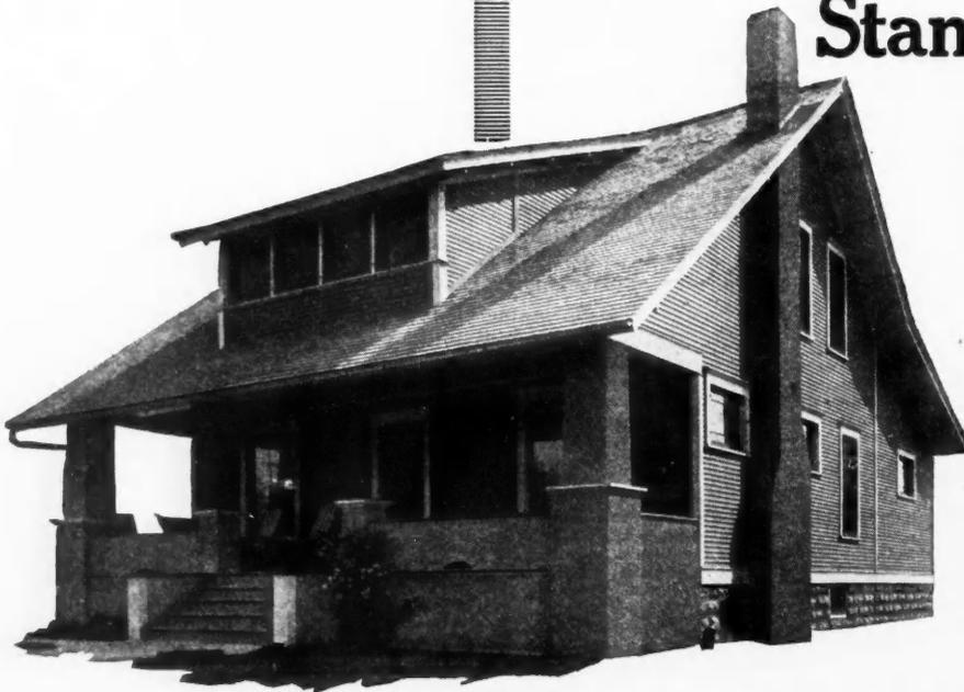
Stucco went into the walls and posts of the porch on this frame house because the builder knew that there was where the wear and tear would be. To make the permanence of the job certain, the stucco was laid on a base of
