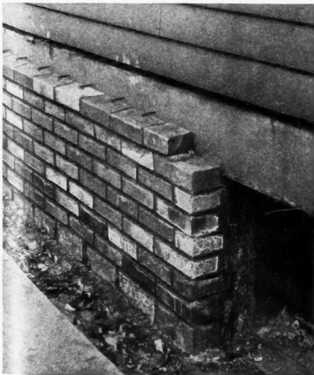
Detail Showing Concrete Foundation for Brick Veneer, Also Method of Tying Brick to Framework of House by Means of 10-Penny Cut Nails.
