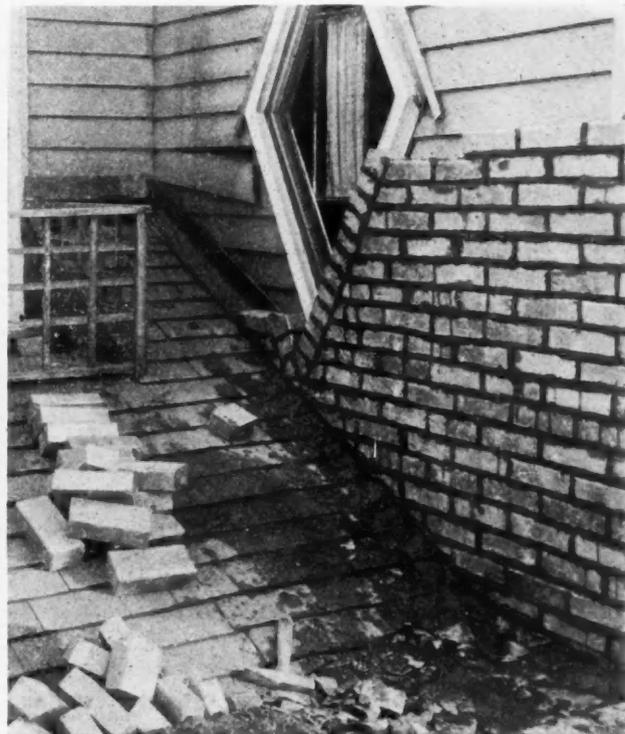
Detail of Supporting Brick Over Porch Roof With 4 by 4 in. Angle Iron Fastened to Joists With Lag Screws.
