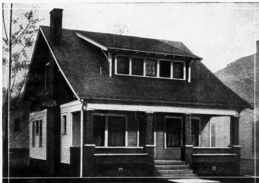
A Practical Little Home Design (No. 6868), Built in Three Different Ways to Show the Use of Three Materials for Outside Walls; Namely, Clapboards, Cement Stucco, and Face Brick Veneer. If Built as Detailed on Opposite Page, the Cost is About the Same for All Three.
