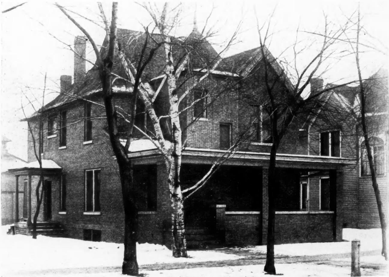
The Remodeled Residence of Mr. Thomson Poor, Streator, Ill. A Veneer of Face Brick Laid Up Without Removing the Clapboards at a Total Cost of \$700, Increased the Selling Value of this Property \$2,500.
