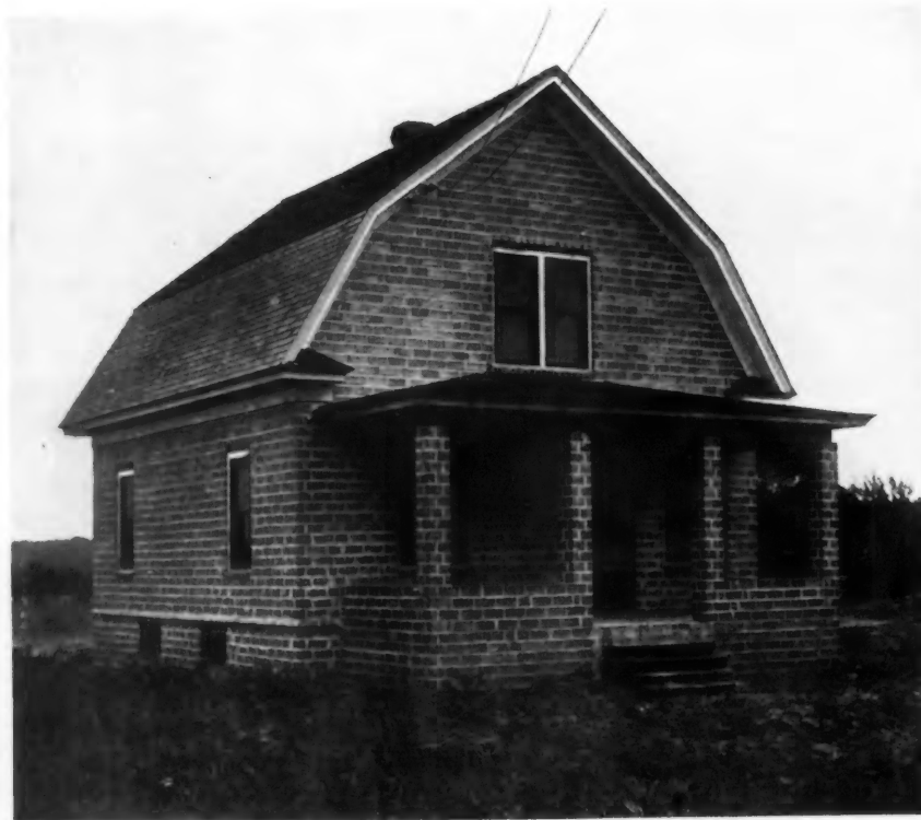
The $1200 House Made of Dark Vitrified Tile Blocks.
