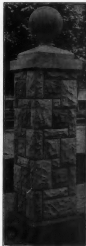
A 20-in. Hollow Pier of Hobbs Broken Ashlar
