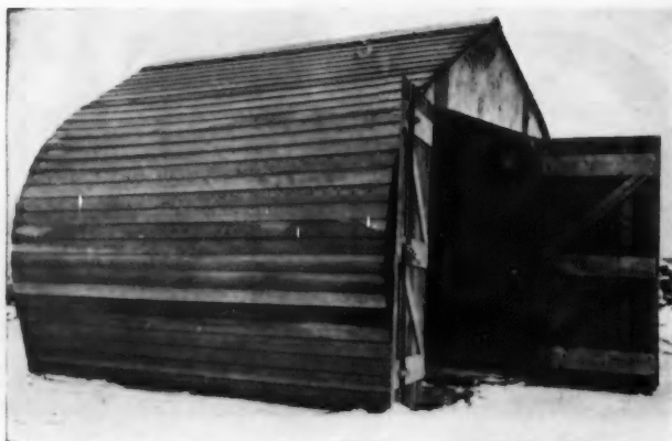
Completed Gothic Roof Garage Built by Chas. R. McPherson.
