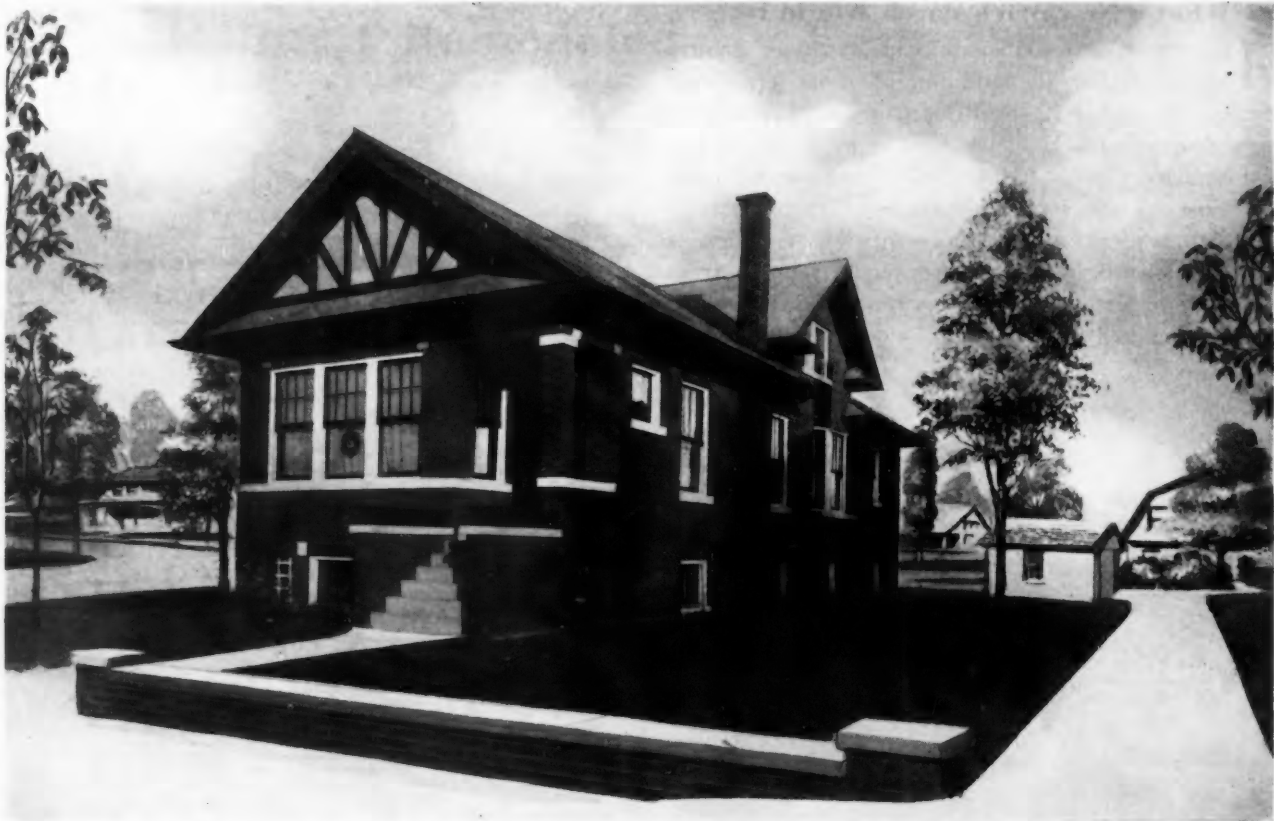
Attractive Brick House Designed for a Narrow Lot. All Walls Are of Solid Brick With the Exception of the Small Portion Under the Main Gable, Which Is of Stucco With Stained Wooden Battens.
