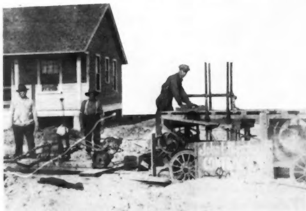
John E. Blanchard (to left) and Two of His Men Operating Power Woodworker.
