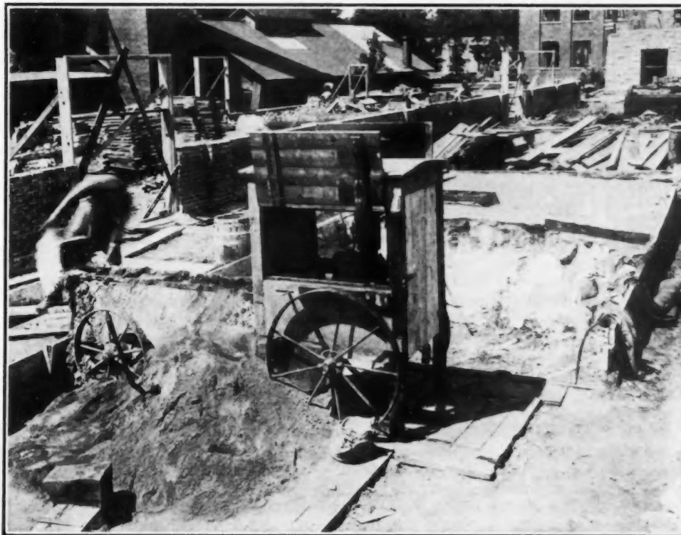
View Showing the Method of Preparing Mortar as Used by the Byers Construction Company of Kalamazoo, Michigan.
