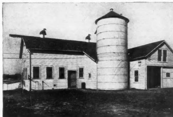
Barn of M. E. Battles, South Euclid, Ohio, which is Equipped with Ventilators of Above Type.
