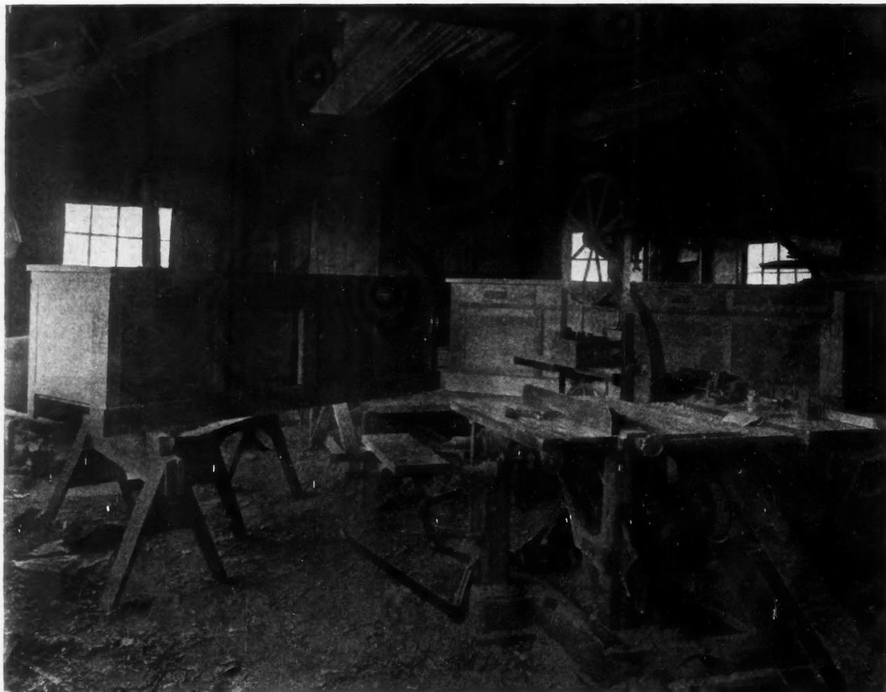
Shop of A. J. Justi, Kingsley, Iowa. Equipped with a Combination Woodworker Consisting of 12-Inch Jointer, 32-Inch Band Saw, Saw Table, Shaper and Borer. Various other attachments can be added to a Universal Woodworker of this type, adapting it for mortising, tenoning, grinding tools, disc sanding, panel raising, etc. A set of store counters and bins just completed by Mr. Justi are shown in the background.
