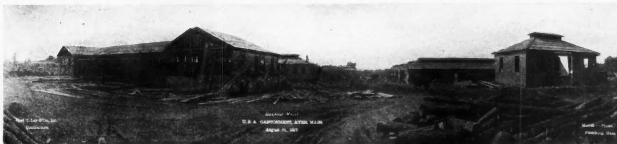
A Typical Building Scene at Camp Devens, showing the hospital unit under construction. The site of this building was marked at first only by a stake bearing its number, 1123. This was used as a guide for the truck drivers in depositing the "Building" in front of it. The figure on horseback is a Squad Chief of Timekeepers.
