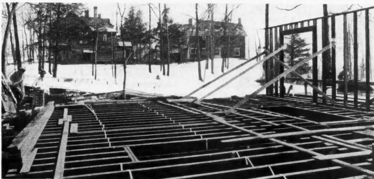
Erecting Metal Lumber Joists and Studs in Winter Weather; Residence of E. H. Fickinger, Yonkers, N. Y., F. W. Conner, Architect.
