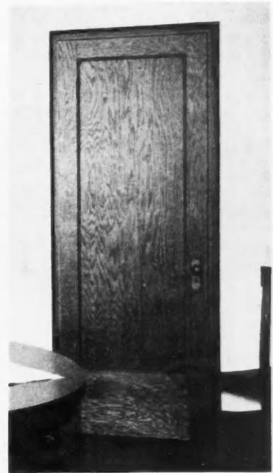
The Appearance of Interior Doors Finished with the Metal Trim is Pleasing and there are no Corners to Catch Dirt or Harbor Vermin.
