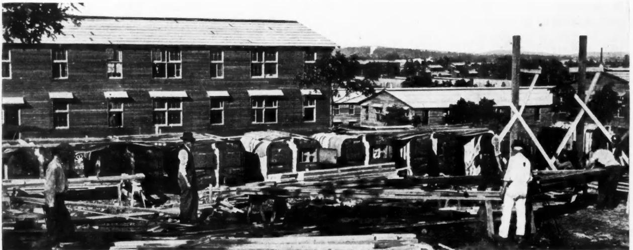
Bollers Have Been Erected in Open Complete, and Afterwards Have a Building Built Around Them. One Such Heating Plant Central for Each Unit or Regiment.
