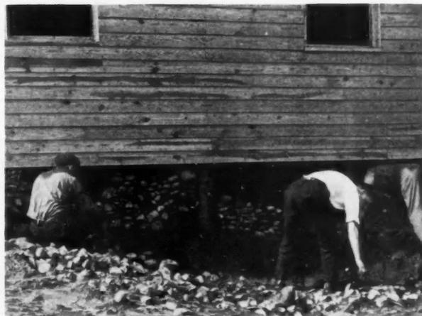
Space Under Buildings Is Filled in if Too Large. If Not, Scarcity and Cost of Labor Were Partly Solved by Leaving Work to be Completed by the Soldiers. Photo Shows Draft Boys Building Wall so That the Winter Winds Will Not Blow Too Cold.
