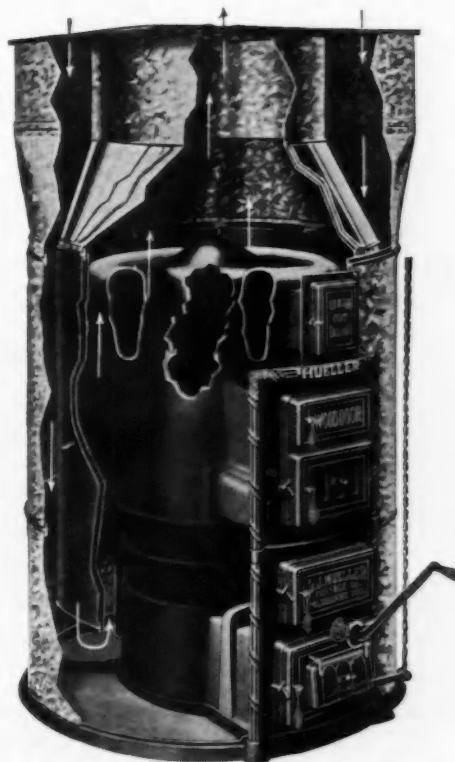
Sectional View of Mueller Pipeless Furnace
