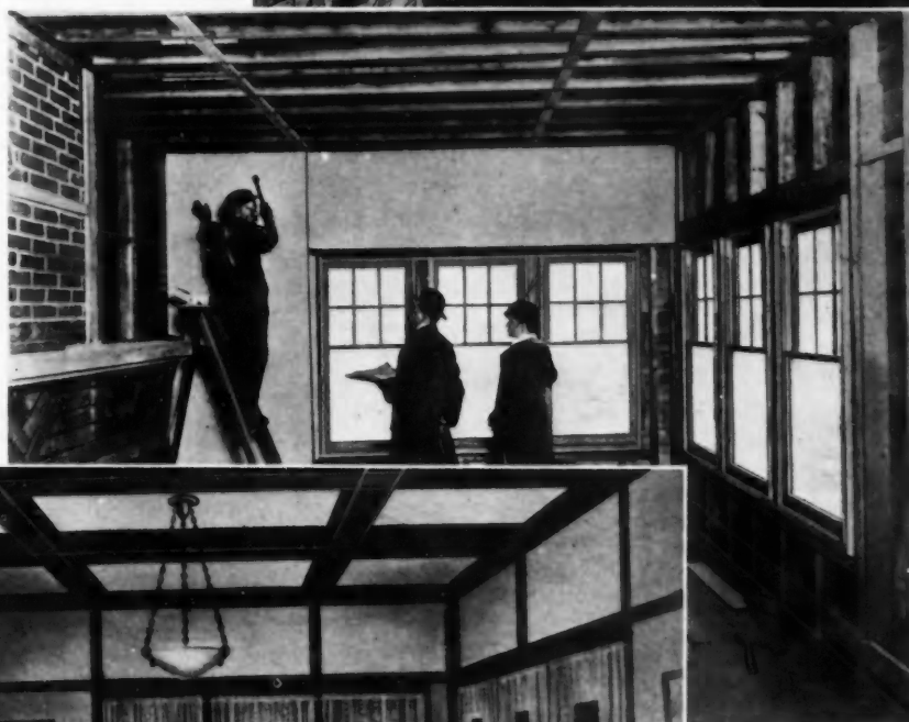
Photo Above — The Wall Board Goes Up Quickly and Easily in Big Sheets.
