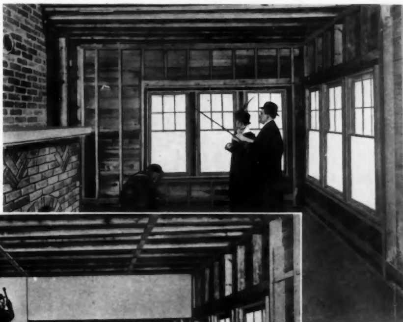
Photo Above — The Carpenter Is All Ready to Begin Putting Up the Wall Board.
