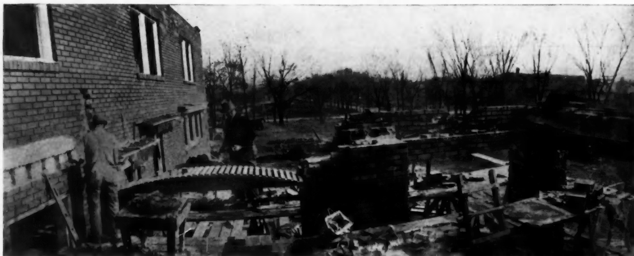
Brick Masons Lay Up Their Walls Carefully and Fashion Strong Arches Over Temporary False Work or Centers.
