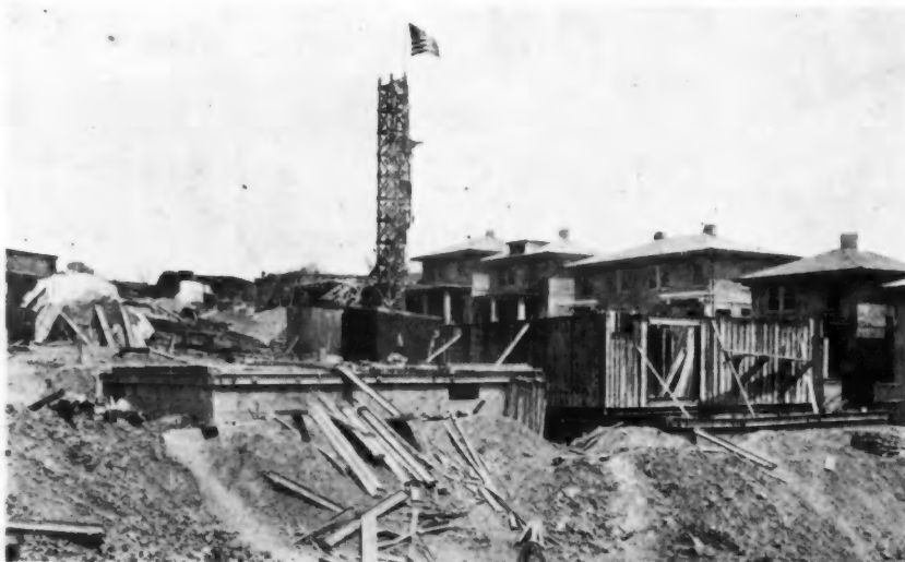
One Hundred Dwellings of Poured Concrete Construction Were Put Up as a Unit at Donora.
