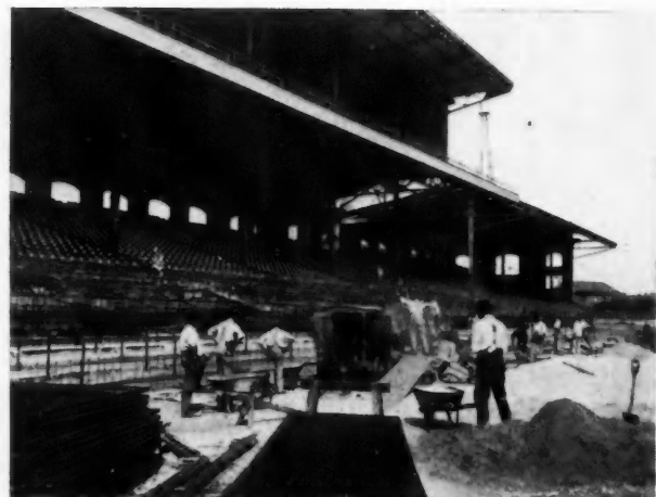
Concreting Gang Putting in 1,000 Additional Box Seats at White Sox Park Before the World's Series.
