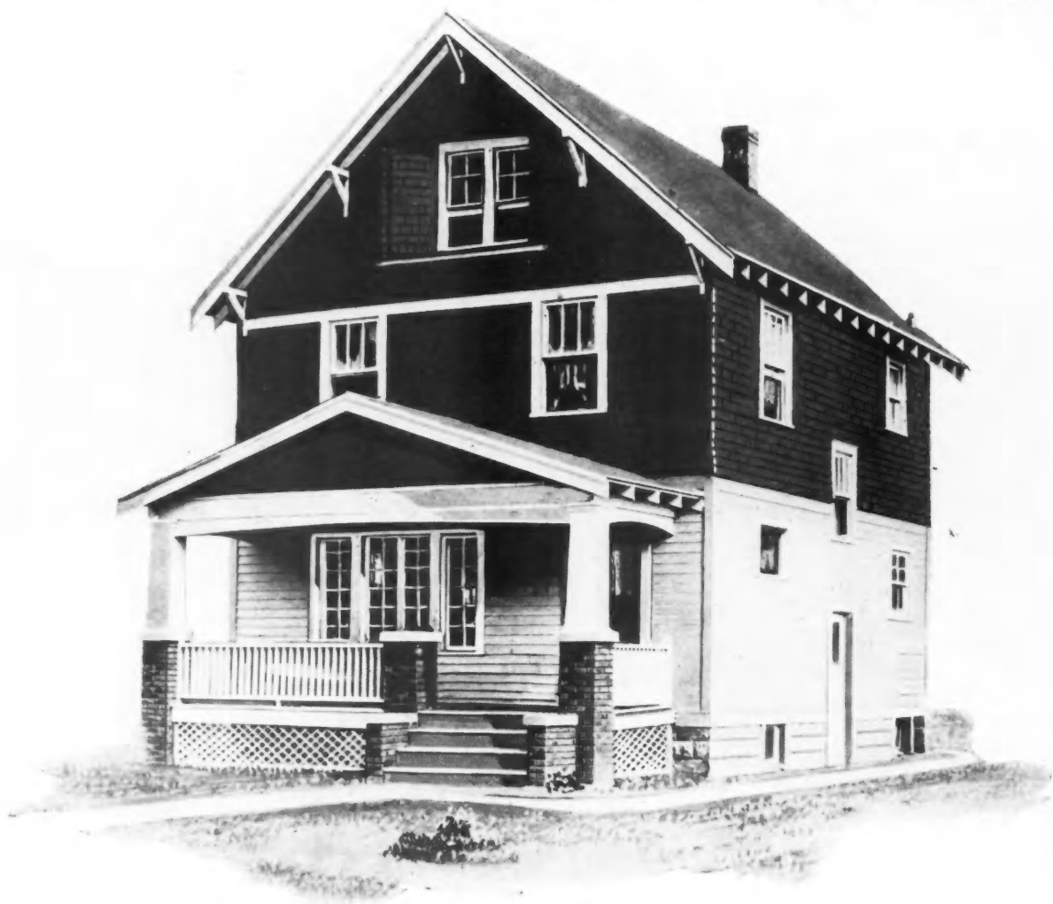
SIX-ROOM FRAME HOUSE. This Design Is Typical of the Homes Built at Firestone Park, Akron, O., a Large Industrial Housing Project that Was Begun Several Years Ago. The House Is of Frame Construction Set on a Concrete Foundation. Its Dimensions Are 22 by 26 Feet, and It Contains Six Well-Arranged Rooms and Bath.
