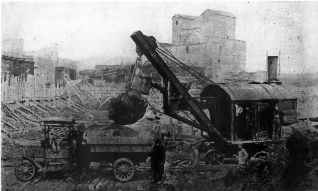
Tons of Dirt and Rock Are Taken from the Building Excavation by the Steam Shovel and Deposited in the Motor Truck. Here Is a "GMC" Truck Waiting for Its Load. Contractors Speed Up Their Work and Do It Economically with Such Motor Trucks.
