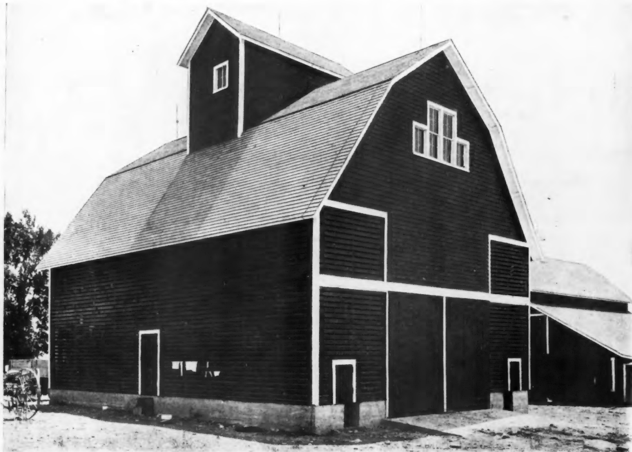
This High Corn Crib Is 40 by 28 Feet, of Frame Construction, with Concrete Foundation and Floor. The Slatted Sides Permit Good Ventilation. It Is Equipped with an Elevator, Making the Putting Away of the Corn Easy and Economical. This Is the Type of Crib That Will House the Corn Crop in Excellent Shape.
