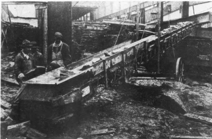
Portable Power-Driven Belt Conveyor Carries Rock Out of a Building Excavation.
