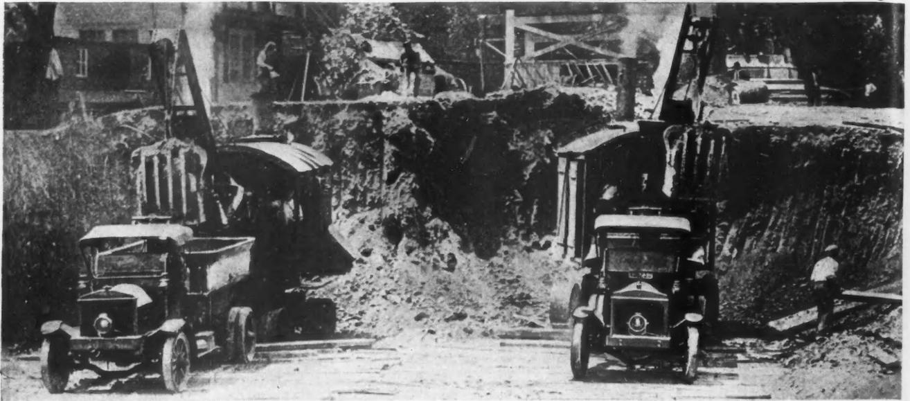
Two "Federal" Trucks at Work Hauling the Materials from the Excavation for the New Annex to the U. S. Treasury Department Buildings, Washington, D. C. Tons of Dirt Were Dug by the Steam Shovels and Carted Away by the Trucks in Preparing for the Building.
