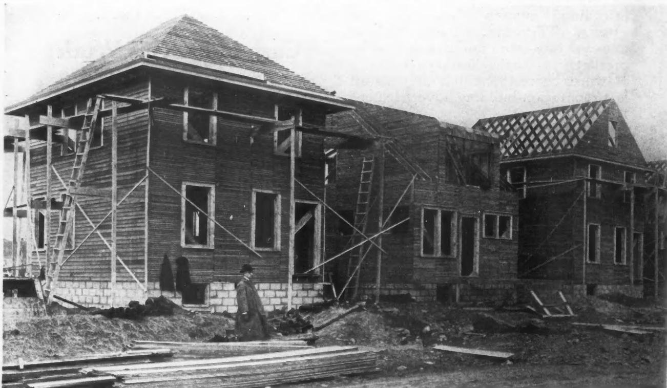
Three Houses Sheathed Ready for the Siding. This Picture Shows How the Sheathing Board Is Applied in Strips, Which Cuts the Labor Cost from 25 to 35 Per Cent
