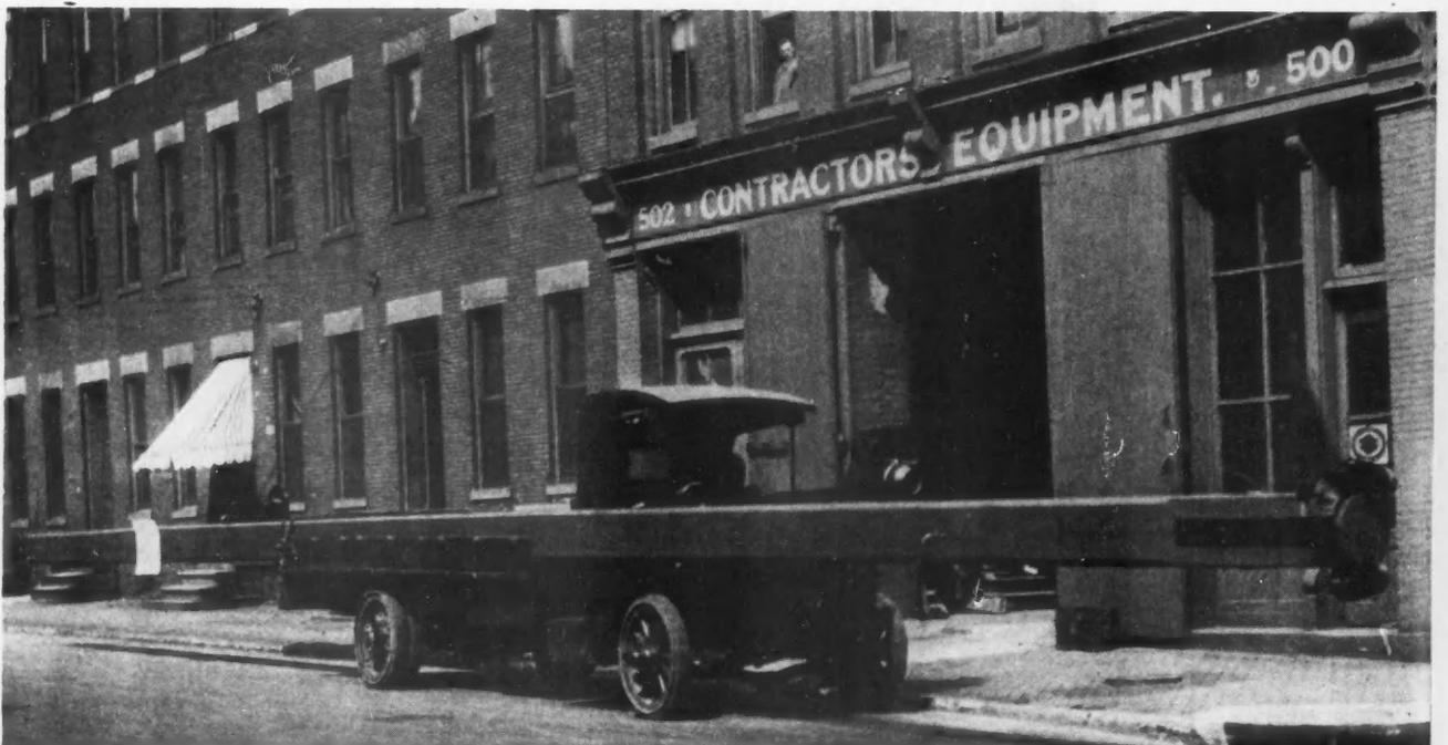
The Special Body "Packard" Truck for Hauling Derrick Masts and Booms by the Beckwith Machinery Co., Pittsburgh, Pa.
