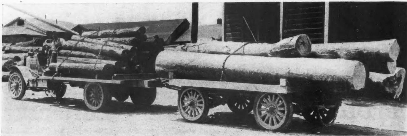
Truck and 3½-Ton "Trallmobile" of the W. J. Steel Lumber Co., Martinsville, Ind. The Trailer Doubles the Capacity of the Truck with Only a Small Increase in the Cost of Operation.
