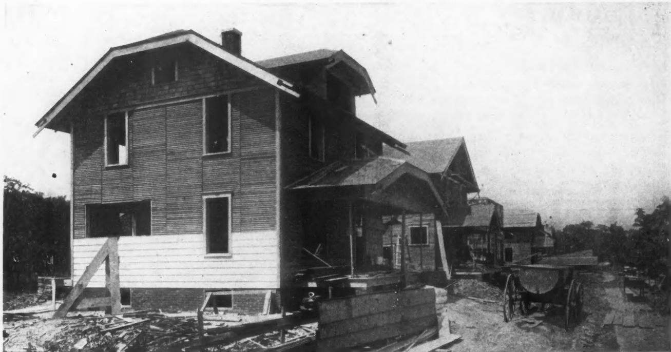
Industrial Housing Project Where Patented Fibre Board, Asphalt and Wood Strip Sheathing Was Used. The House in the Foreground Has Been Sheathed, Shingle Siding Is on Under the Eaves and Board Siding Is in Place Above the Sill Course.
